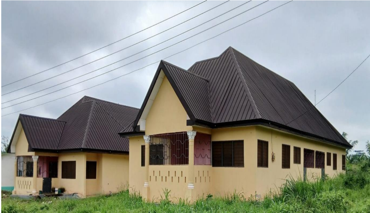
Completed the Construction 4 Unit 2 bedroom staff quarters at Kenyasi No.1
