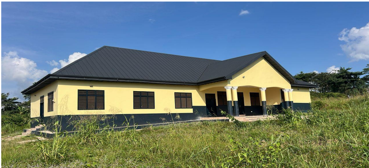
Construction of District Police Headquarters at Kenyasi No.1
