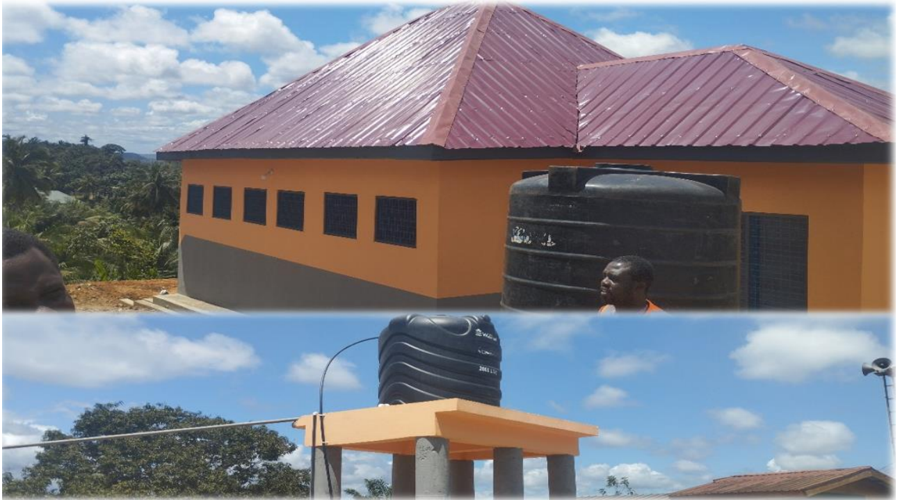
Completion of 12 Seater Water Closet at Bokoro
