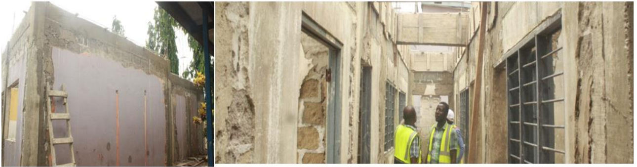
Rehabilitation of the MPCU Block
