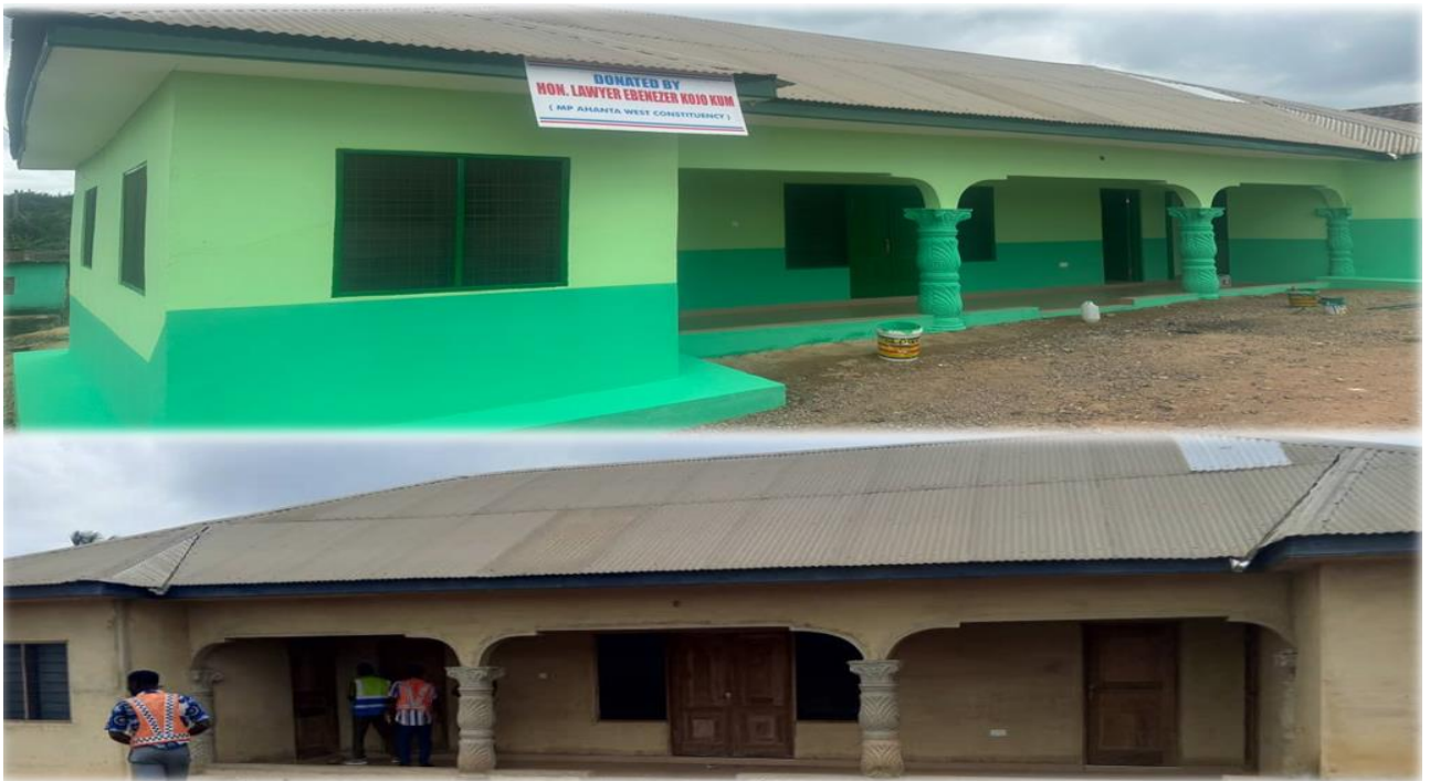
Completion of CHPS Compound at Mpatase
