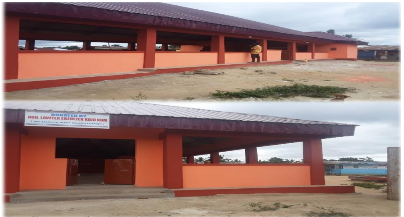
Completion of Community Centre at Fasin - MPCF
