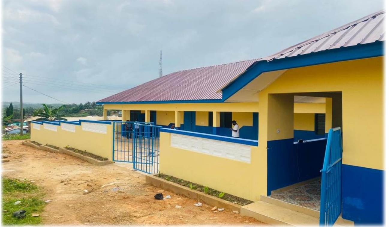
Rehabilitation of 3 Unit Classroom block at Akwidaa
