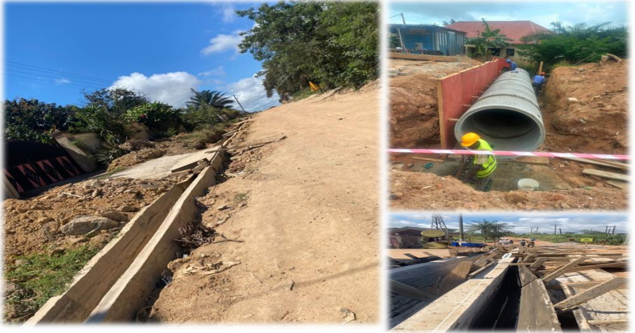
Construction of Bituminous Seal of Apowa Junction (TUC Estate Rd) - GSCSP
