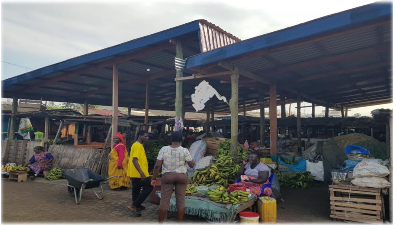
Construction of 1No. Market Shed at Agona Nkwanta market
