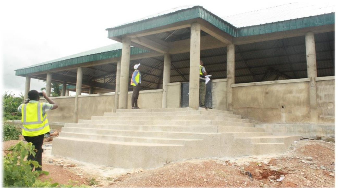
Construction of Community Centre at Egyam
