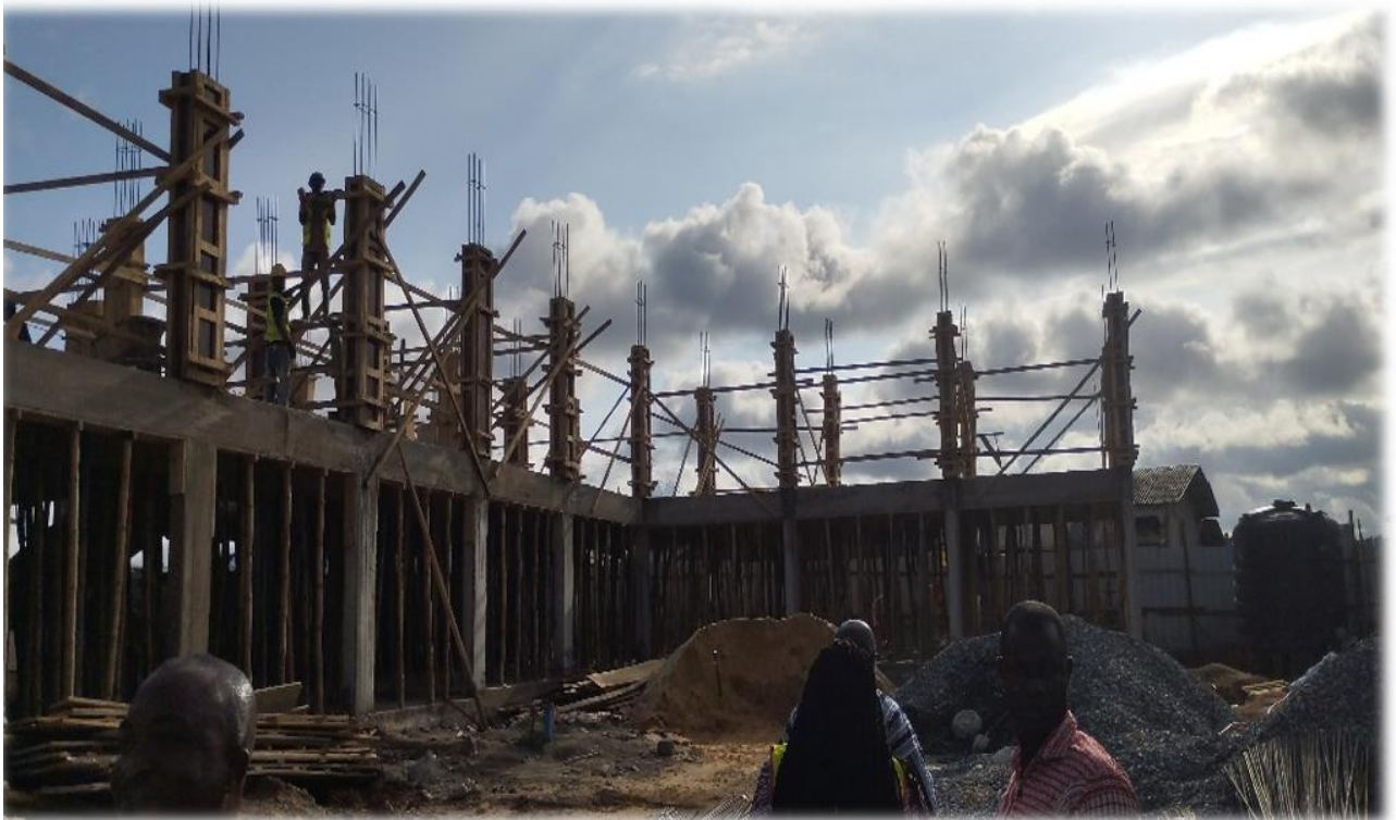
Construction of 50.No. Lockable Shop with Boreholes at Agona Nkwanta Market -
