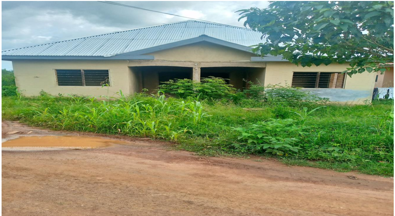
Construction of 1No 2Unit Semi-detached Nurses Quarters- Dadieso
