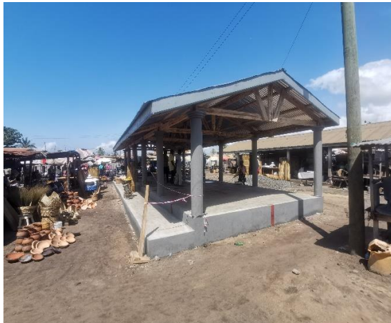
Constructed market shed at Aflao market
