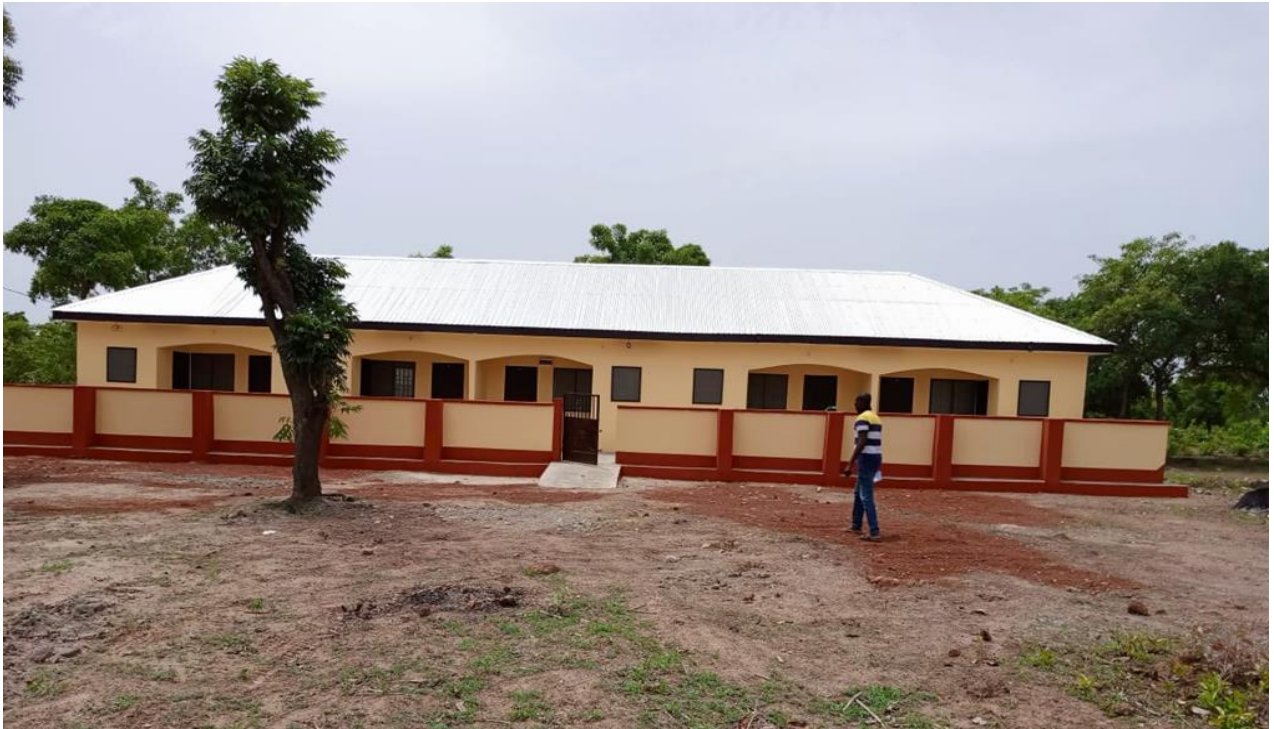
Constructed and Furnished 1No. 5-Unit Teachers Quarters at Jenbob (SOCO)
