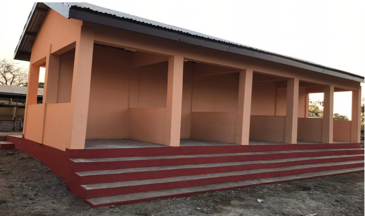
Constructed 10-Unit market stalls at Wechiau(SOCO)
