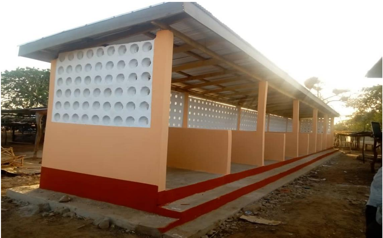
Rehabilitated 5-Unit market Stalls at Tanvaare (SOCO)
