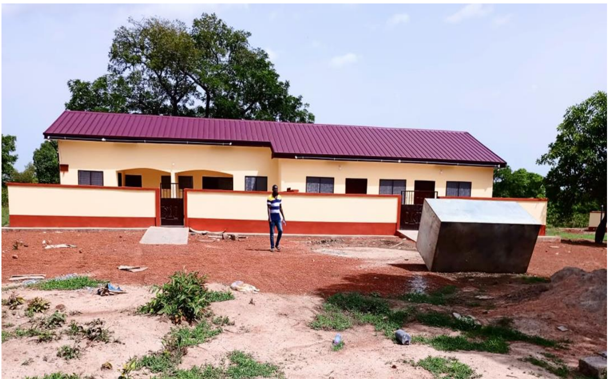
Constructed and furnished 1 No. CHPs compound at Batunuuriyiri(SOCO)
