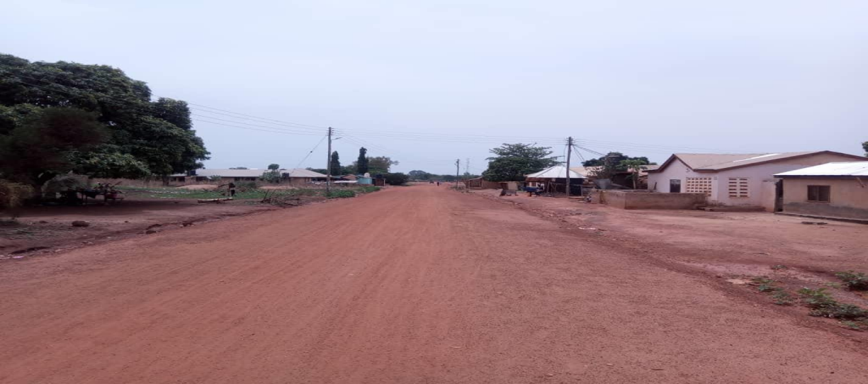
Figure 3. Bolga High tension link road
