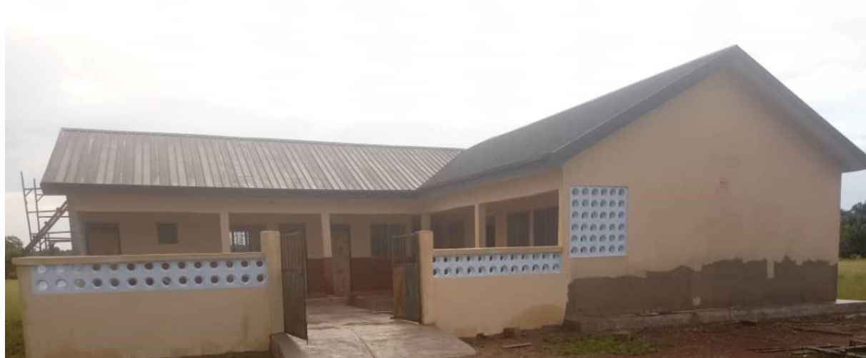
A 2-unit KG Block at Zambo Baagaun FUNDING SOURCE: WORLD BANK (SOCO)
