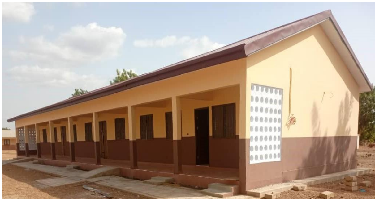
A 3-unit Classroom Block at Kuoli FUNDING SOURCE: WORLD BANK (SOCO)
