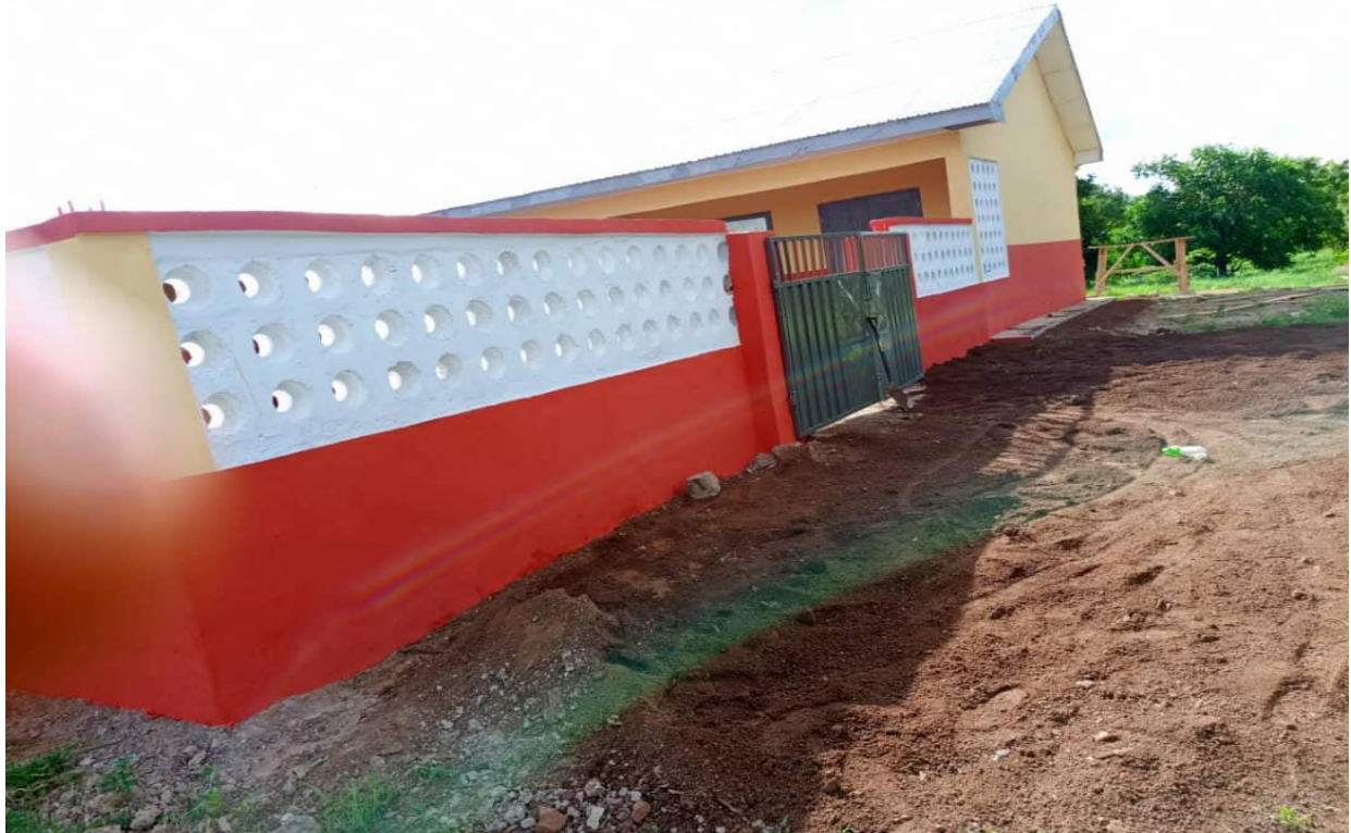
Construction of KG Block at Bussie-Moyiri
