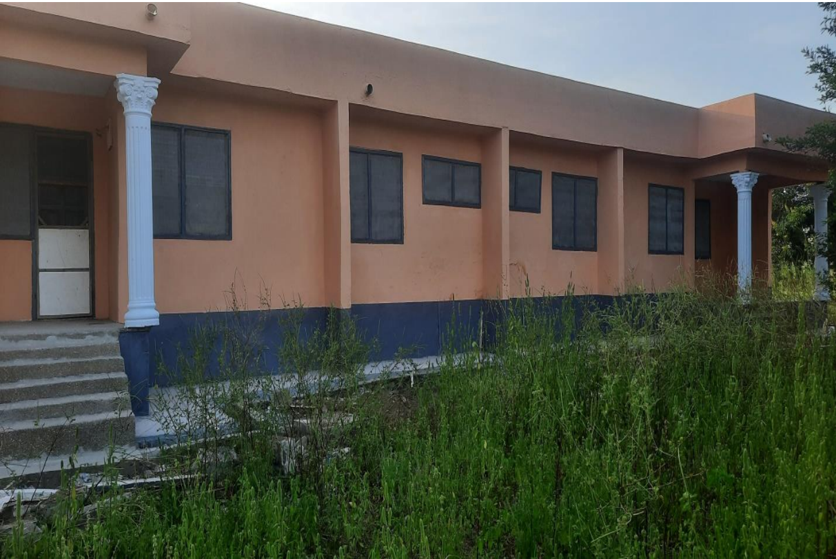
Renovated 2no. semi-detached health quarters at Sandema under SOCO
