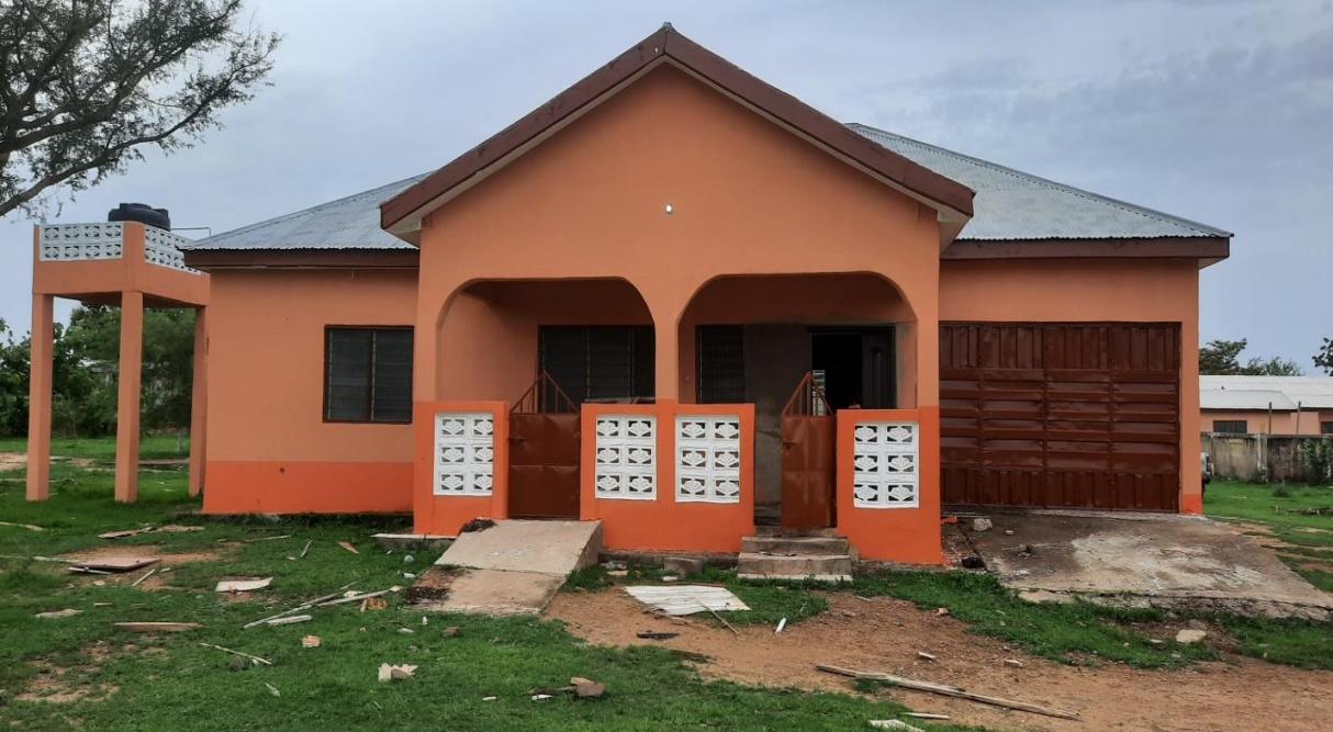
Renovated Magistrate bungalow at Suwarinsa under DACF
