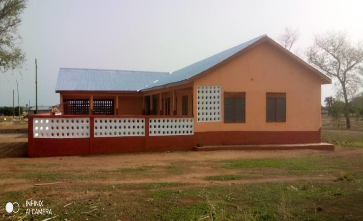
Renovated Wiaga Chiok Atidiok KG school block under MPCF
