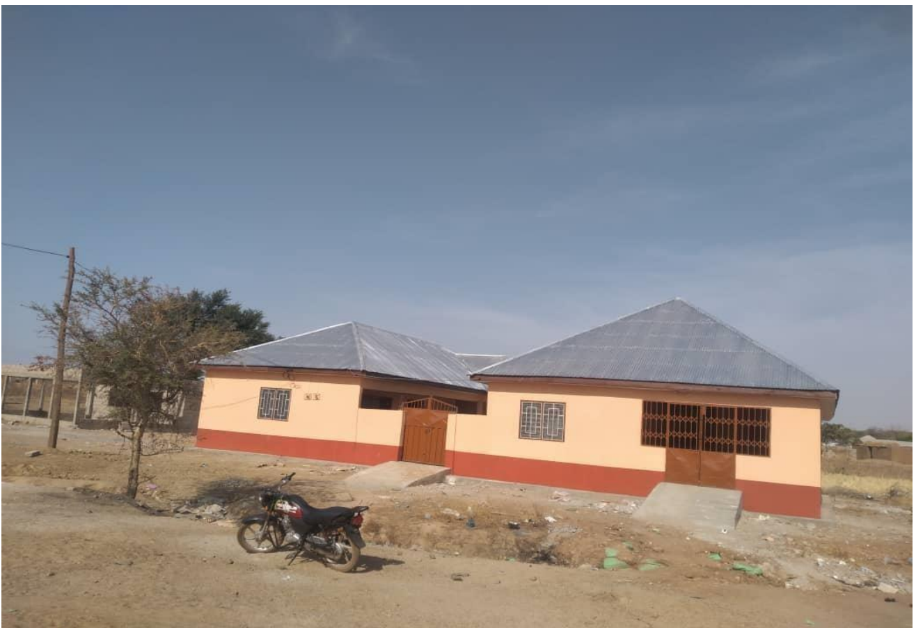
Construction of 1No.CHPS Compound at Kpalugu with furniture
