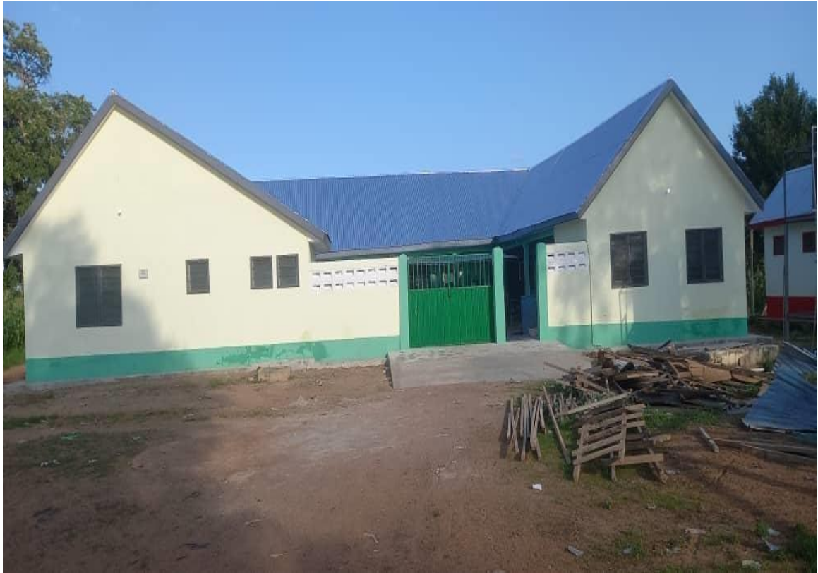
Construction of 1NO.
