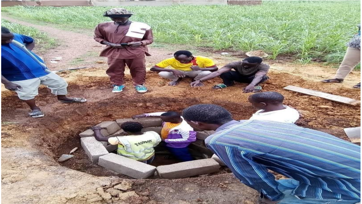
CLTS - Training of Artisans on Latrine Construction at Tegbilla
