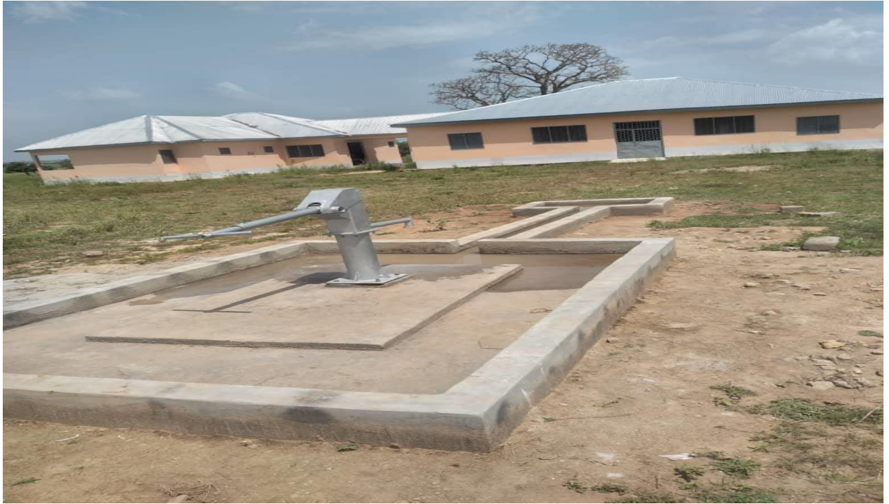
Drilling & Construction of 4No. Boreholes fitted with Hand Pumps at Bakanga, Barabogo, Manga, and Sakpari
