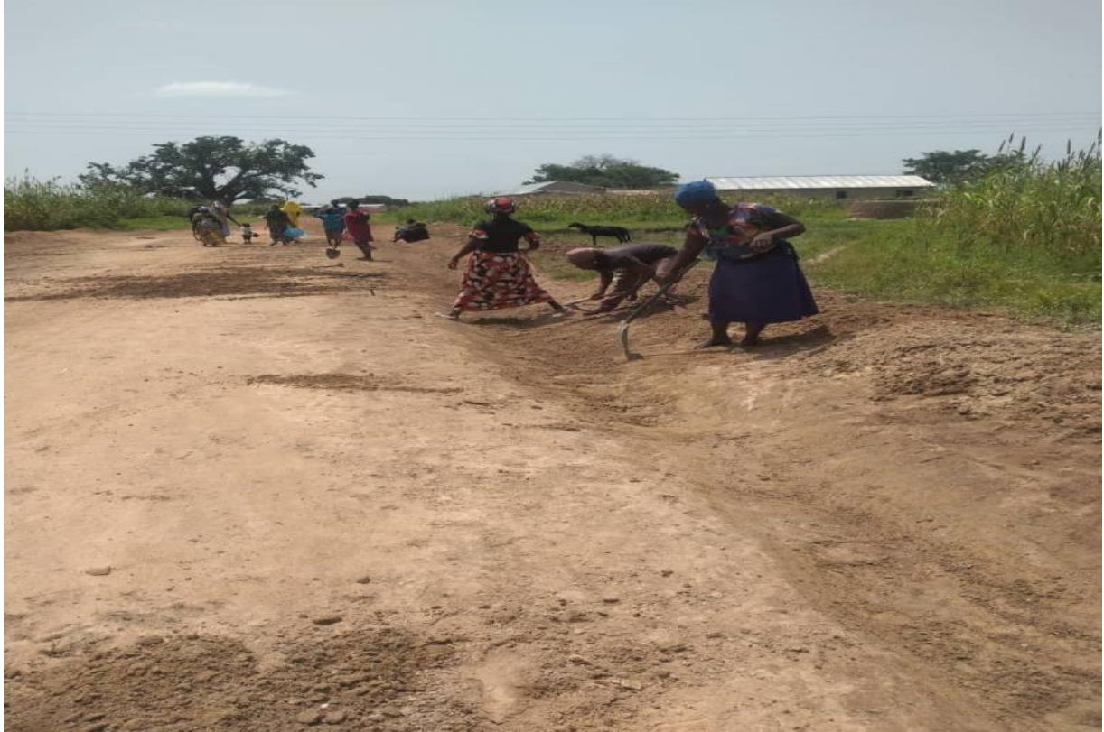
Rehabilitation of Nayoko No.2 - Goore Clinic Feeder Road (5.5Km)
