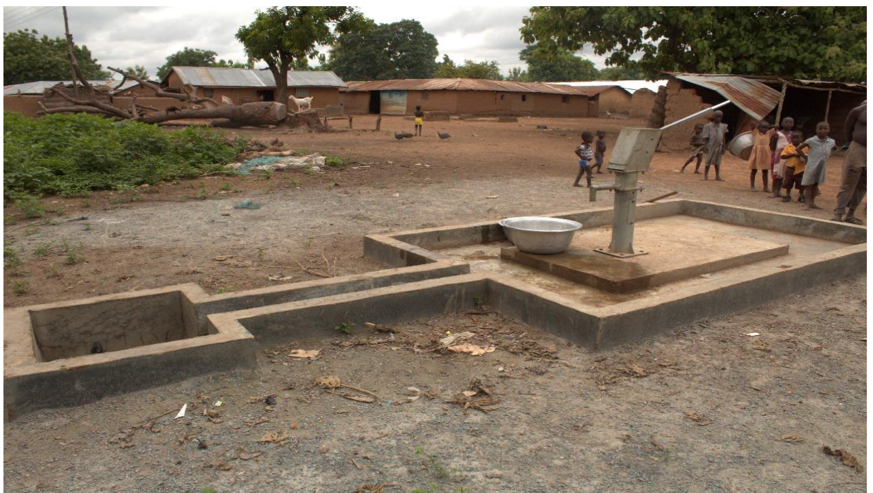
SITED AND DRILLED 1 NO. BOREHOLE FITTED WITH HANDPUMP AT OJAGANDO
