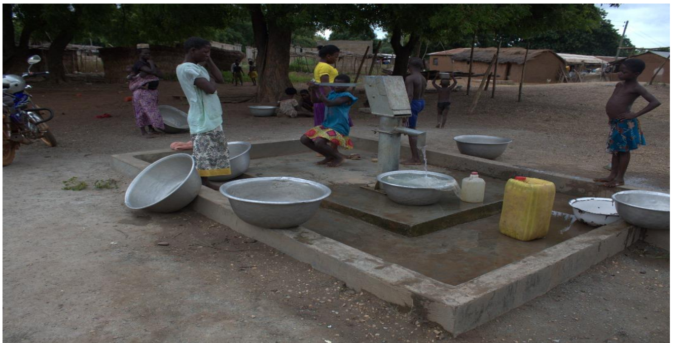
SITED AND DRILLED 1 NO. BOREHOLE FITTED WITH HANDPUMP AT PIBILA
