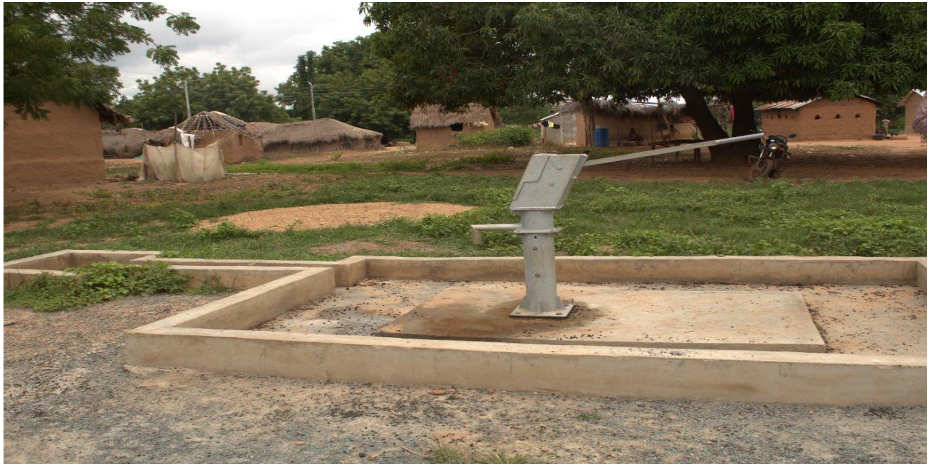
SITED AND DRILLED 1 NO. BOREHOLE FITTED WITH HANDPUMP AT MOLA NO.2
