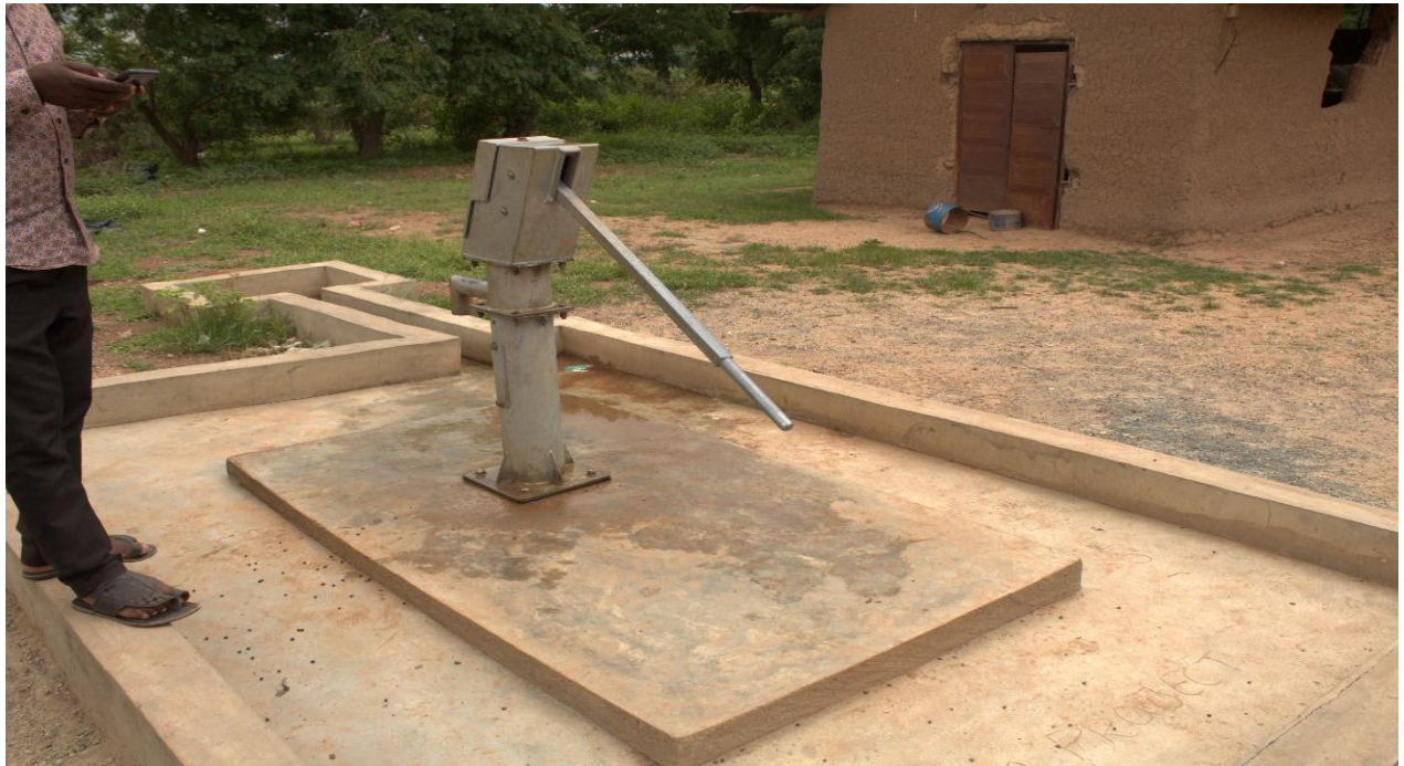
SITED AND DRILLED 1 NO. BOREHOLE FITTED WITH HANDPUMP AT OJAGANDO
