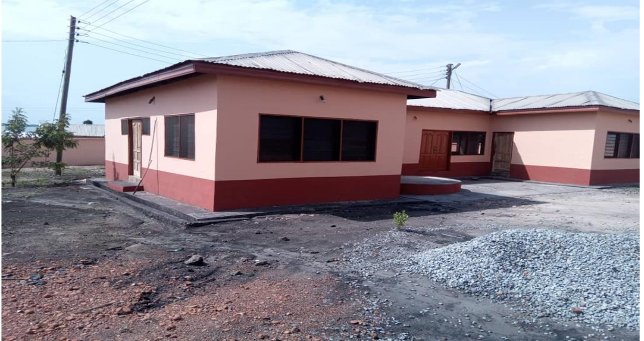
5. Constructed 1 No. 3 unit classroom block with ancillary facilities at Tokuroano
