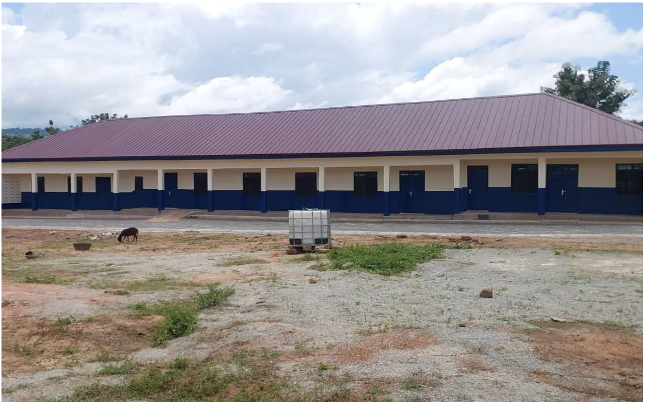
1. Constructed and furnished a theatre block at Dambai health centre
