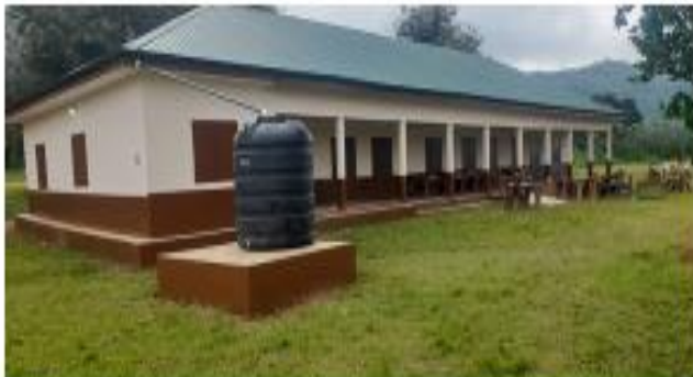
Rehabilitated a 3-unit classroom block at Likpe Mate R.C JHS - DACF
