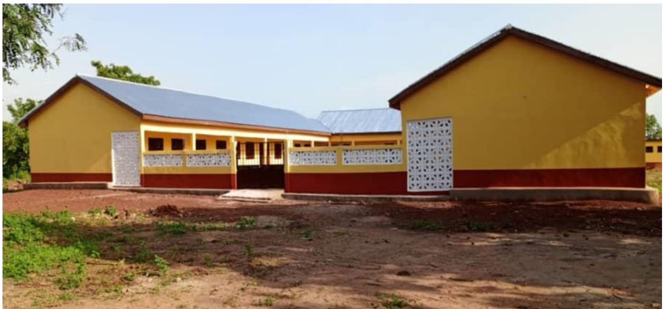
CONSTRUCTION AND FURNISHING OF 1NO. 6 UNITS CLASSROOM BLOCK AT POALARIDO (COMPLETED) BY SOCO
