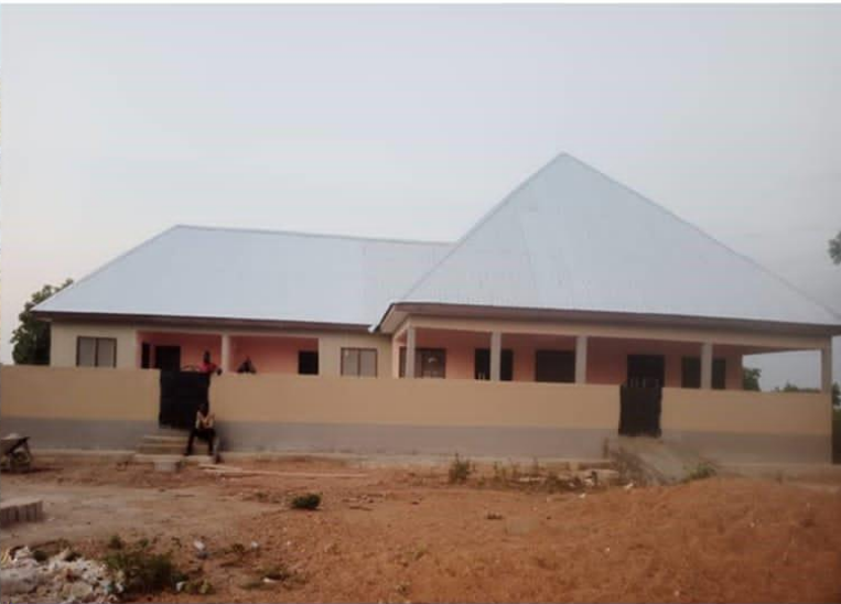
CONSTRUCTION OF 1NO. CHPS COMPOUND AT NKPANGINI BY SOCO
