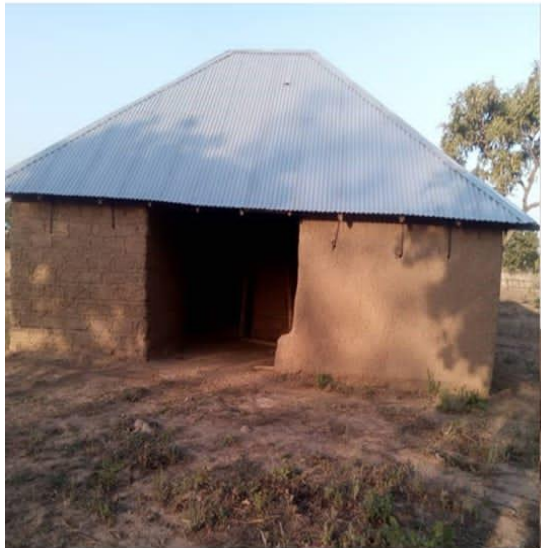
COMMUNITY INITIATED CHPS COMPOUND AT NKPANGINI
