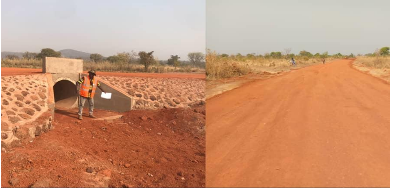
REHABILITATION OF 7KM CHAKUDO – JAYUNDO FEEDER ROAD (COMPLETED) BY SOCO
