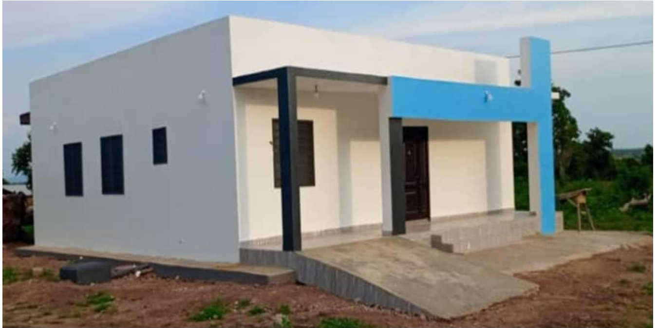
CONSTRUCTION OF HEALTH CENTER AT NAHUYILI (COMPLETED) BY MPCF
