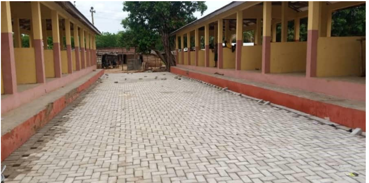
CONSTRUCTION OF 3NO. 20 UNIT MARKET SHED AT SHEINI (COMPLETED) BY SOCO
