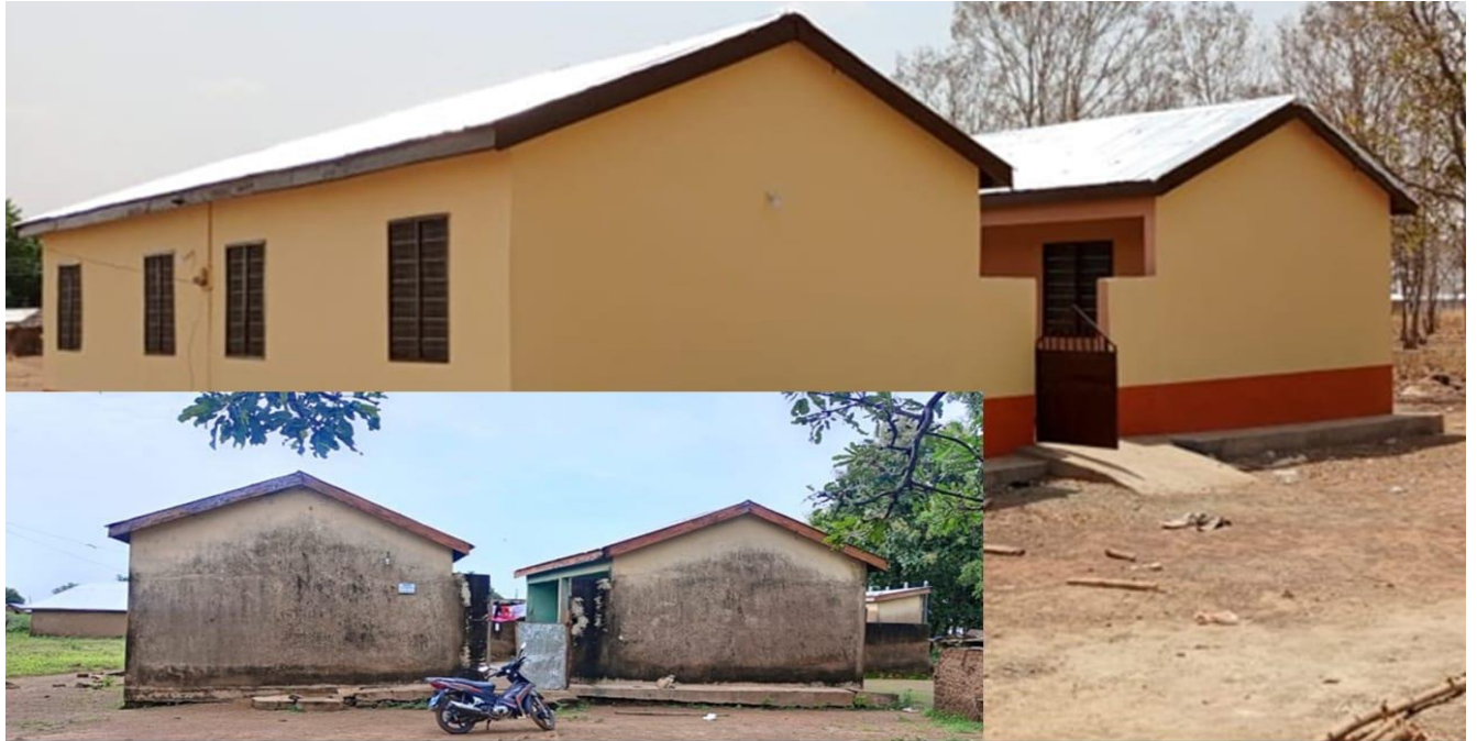
REHABILITATION OF 6 BEDROOM TEACHER'S QUARTERS AT SANGULI (BEFORE & AFTER) BY SOCO
