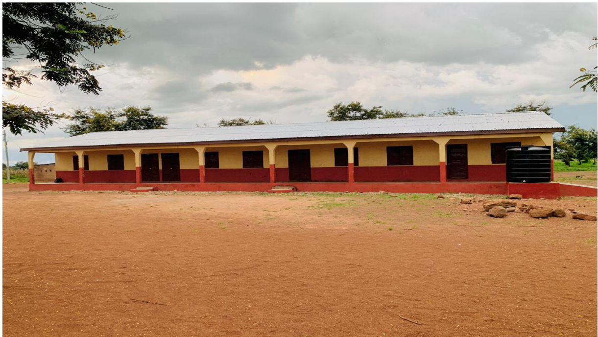
Figure 1: Rehabilitated 1 No. 3-Unit Classroom Block at Sahakpalugu (Completed)
