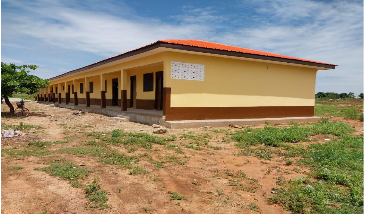
1No.3unit classroom block with ancillary facilities at Tojing
