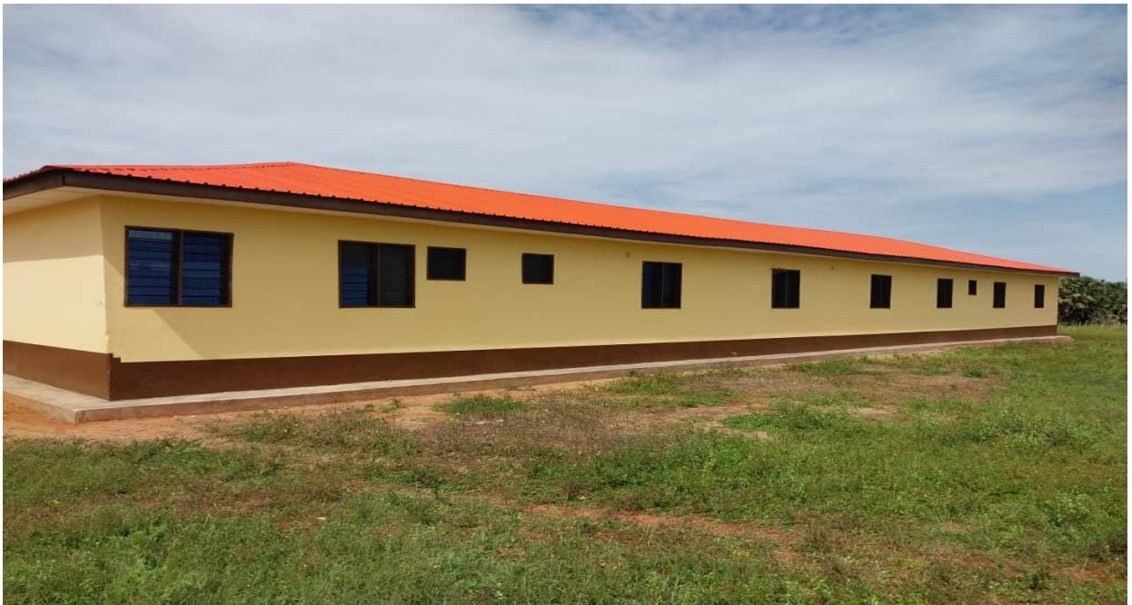
1No. 3unit classroom block with ancillary facilities at mayeem
