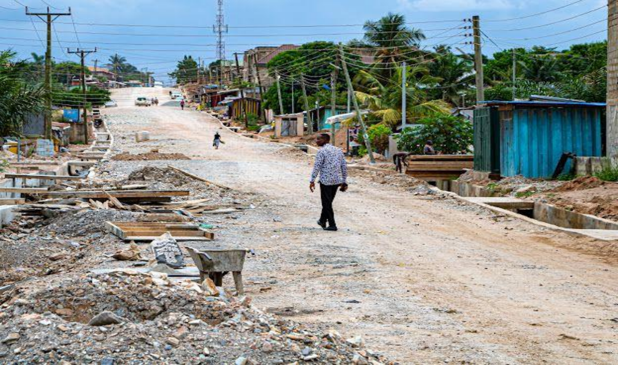
Picture 3: PARTIAL RECONSTRUCTION OF ISREAL TO PENTECOST UNIVERSITY ROAD
