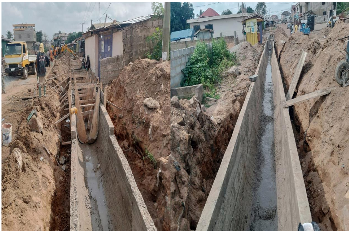
Picture 5: CONSTRUCTION OF 0.9M U-DRAIN AT ABLEKUMA ABEASE
