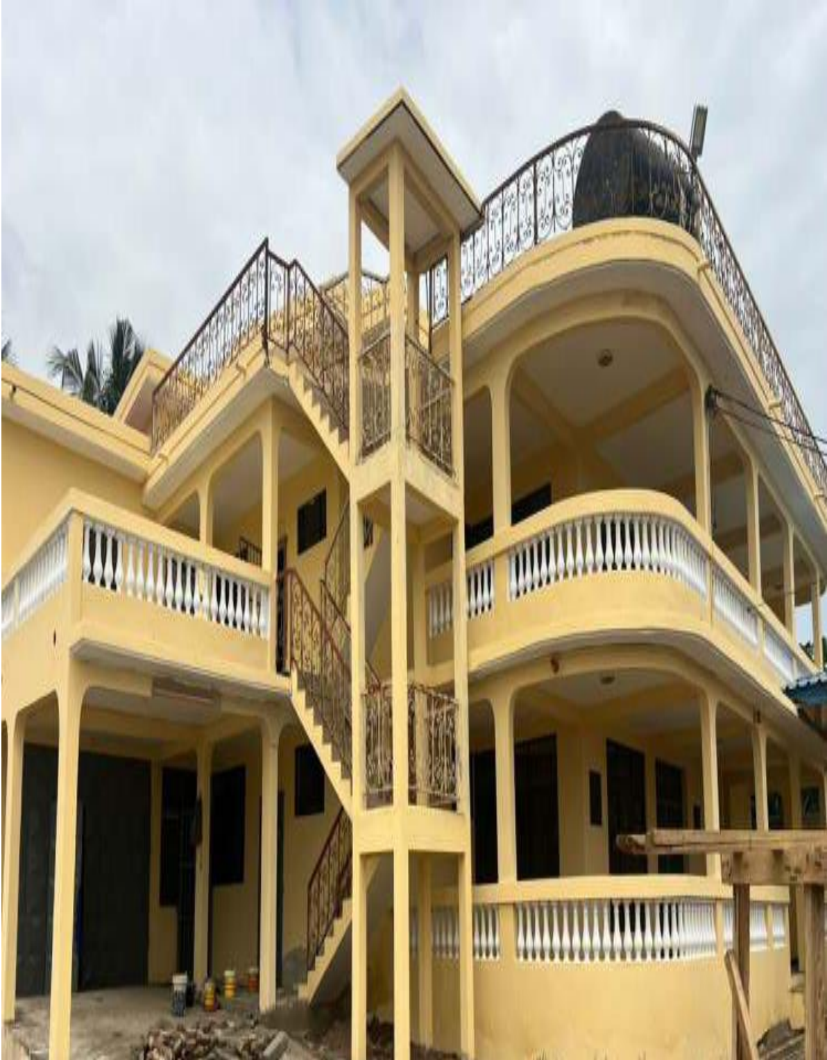
Picture 8: RENOVATION OF OFFICE ANNEX AT AGAPE
