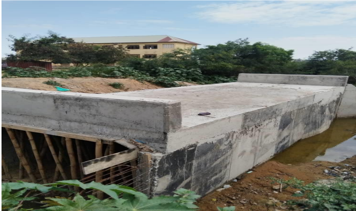
Picture 4: CONSTRUCTION 3.5Mx2.5M BOX CULVERT AT ANTI-AKU
