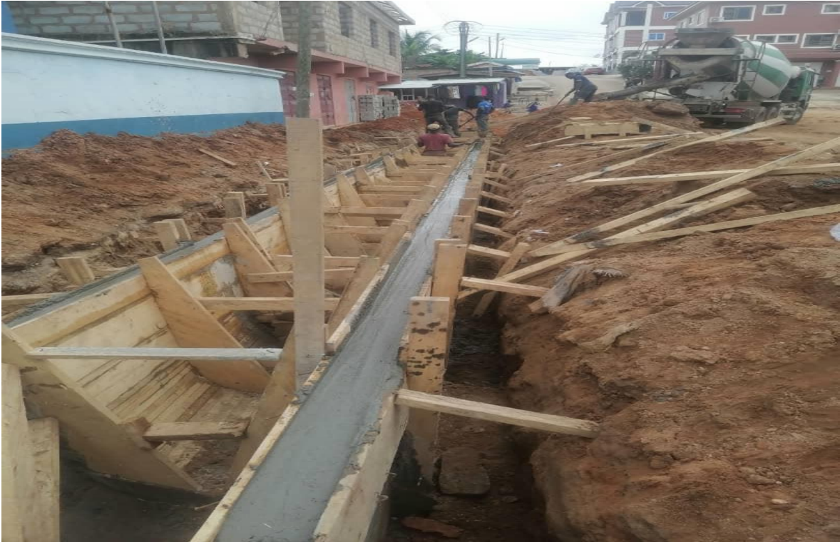
Picture 6: CONSTRUCTION OF 0.9M U-DRAIN AT KWASHIEBU
