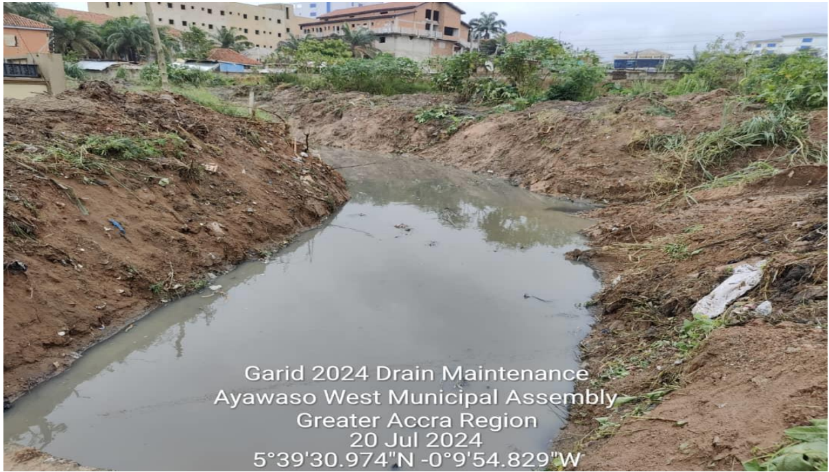
Desilted 850m drains at Mempeasem
