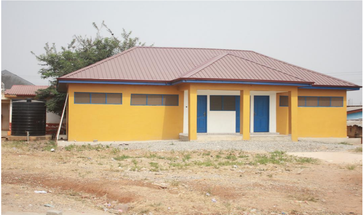
Constructed 14-Seater WC Toilet Facility and overhead Water Reservoir at Abelenkpe Basic Primary School
