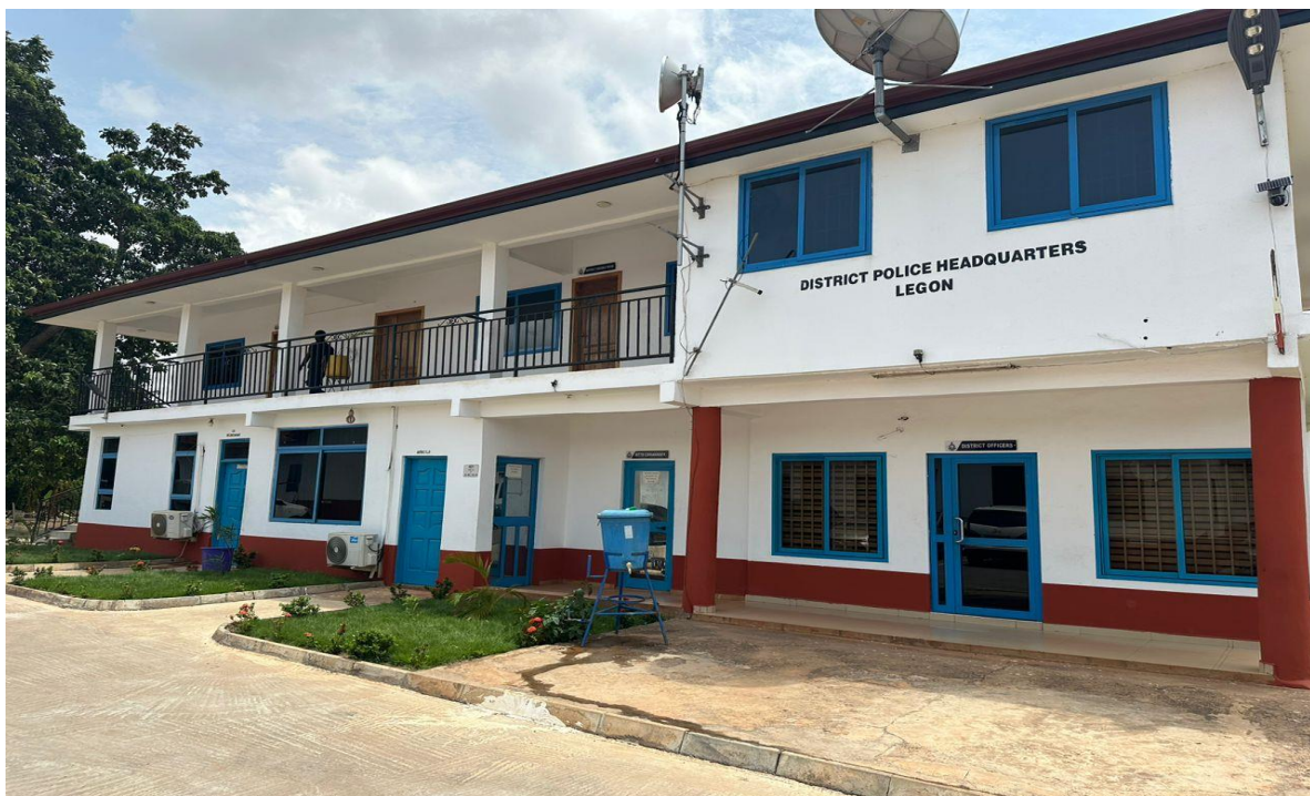
Painting works at Painted Legon Police Station
