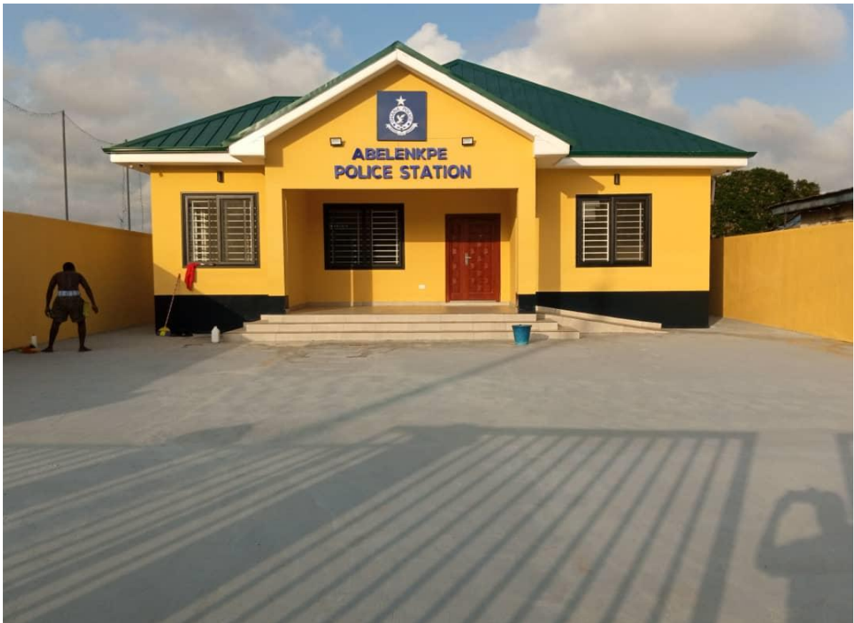
Constructed a Police Station at Abelenkpe
