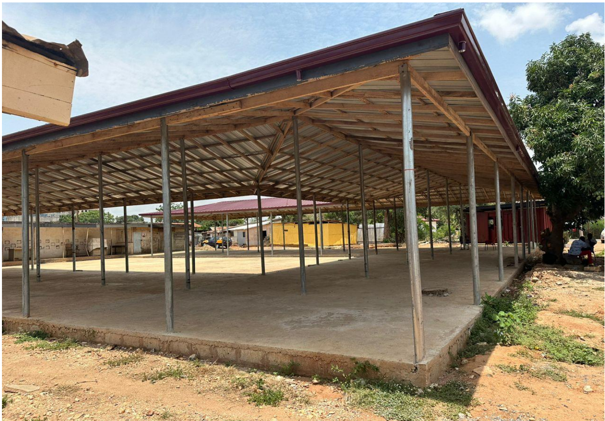
Constructed a community center at Legon Staff Village
