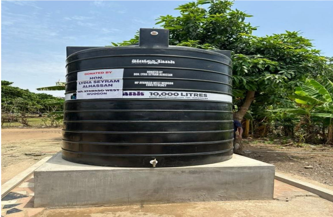
Constructed 5No. Mechanized Boreholes with Water Tanks within the Municipality
