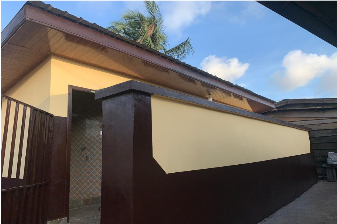
Constructed 6No. WC Seater toilet facility with washroom at Santana Market
