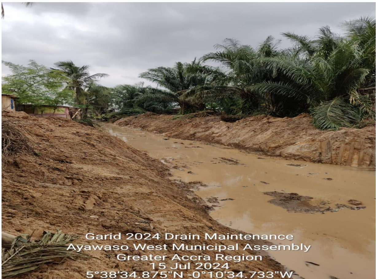
Desilted 830m Okponglo Township drains
