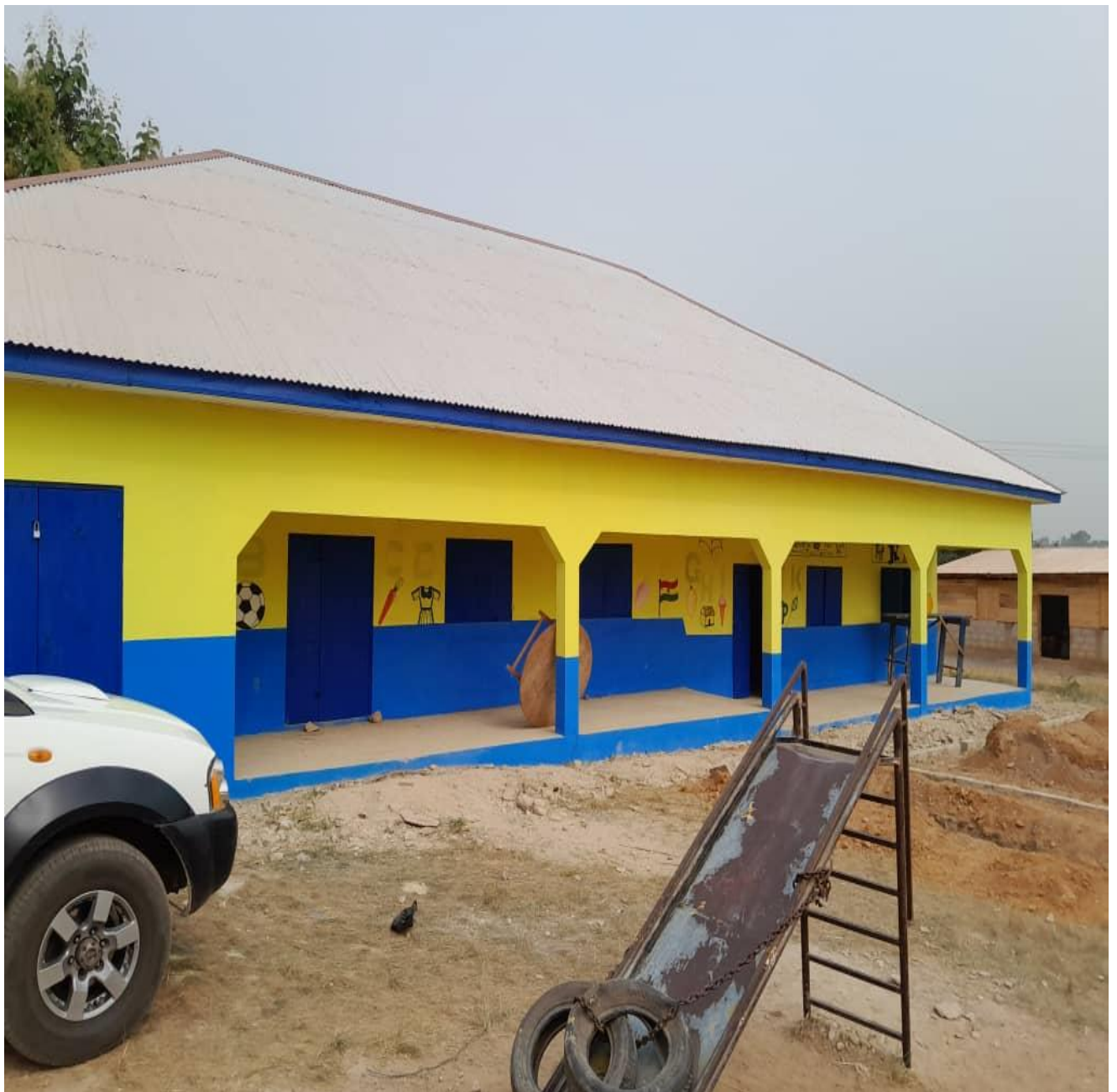
Renovation of 1No. KG Block at Asuokaw Methodist KG
