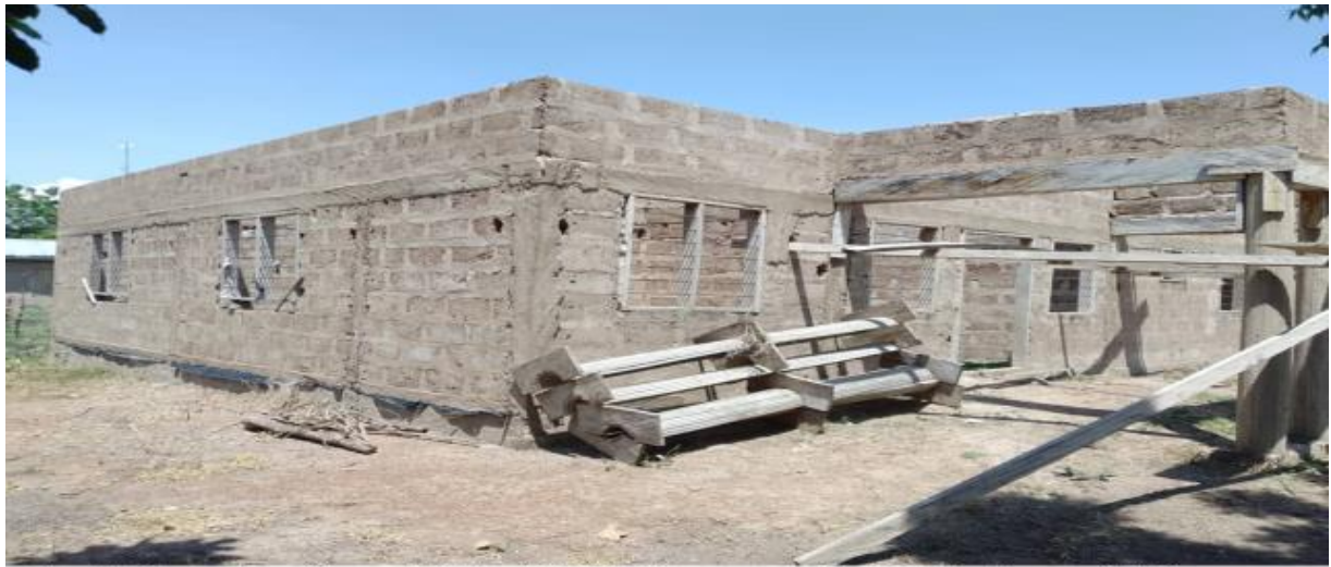
Fig 7: Construction of 1 No CHPS Compound at Batorkope (65% Complete)
