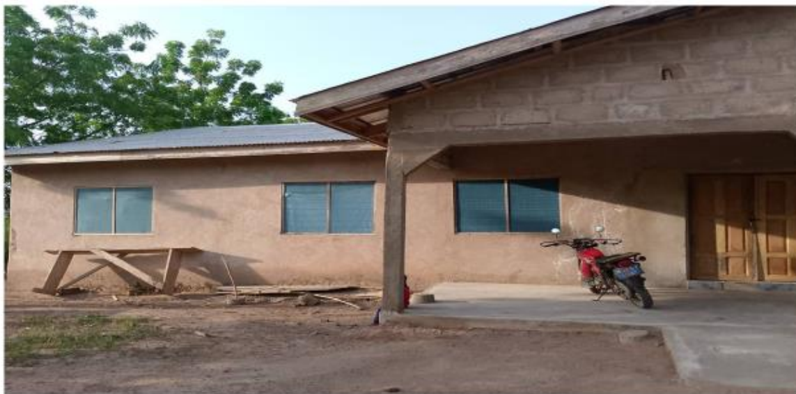
Fig 8: Construction of 1 No. CHPS Compound at Kokrobuta (85% Complete)
