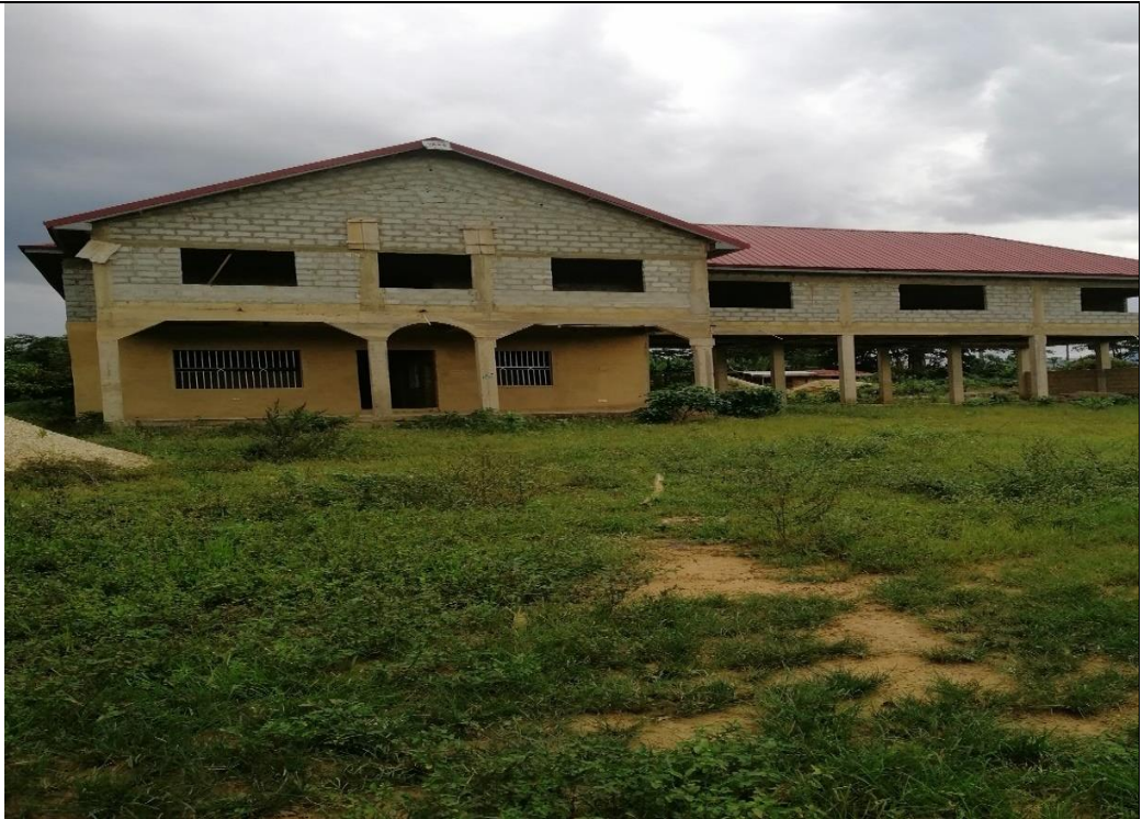
Construction of District Fire Service Office Area at Akyem Kwabeng
