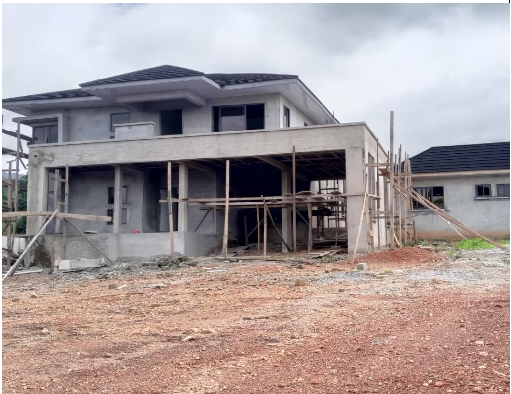
Construction of DCE's Residence at Bomaa
