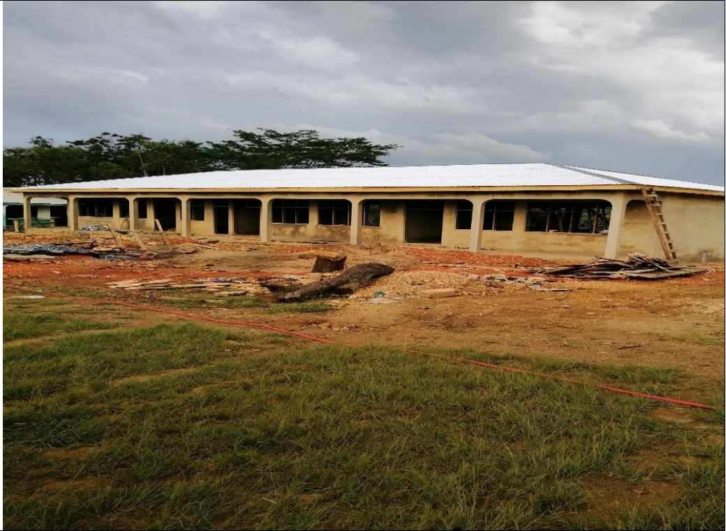
Construction of 3-unit classroom block at Anglican JHS at Akyem Kwabeng
