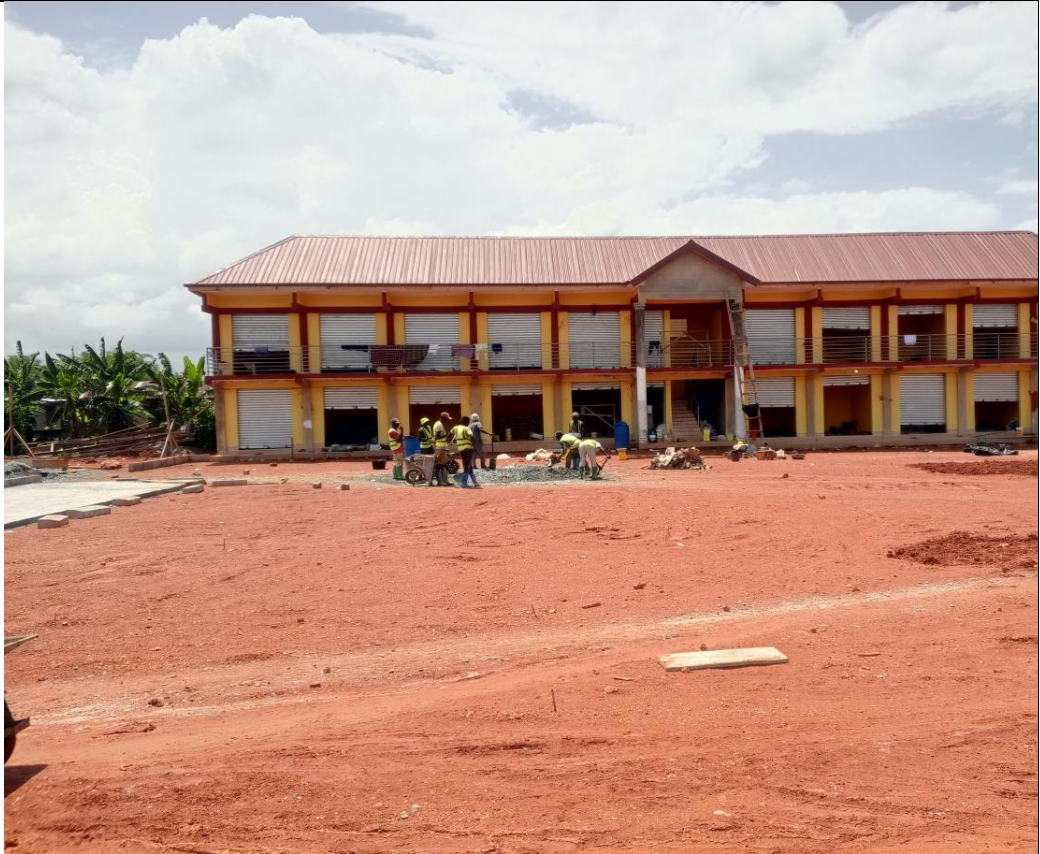
Construction Of 22-Unit Lockable Stores, Stalls And Shed At Akyem Akropong
