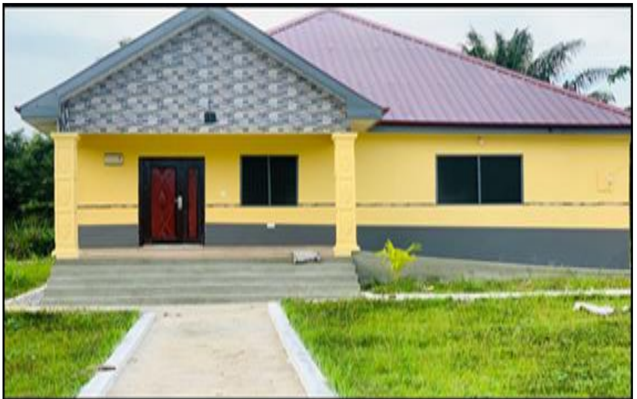
Completion and operationalization of Siawkrom & Teshieman CHPs Compounds.
