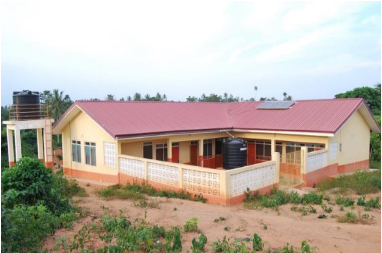
NEW KINDERGARTEN BLOCK AT KOKOADO
