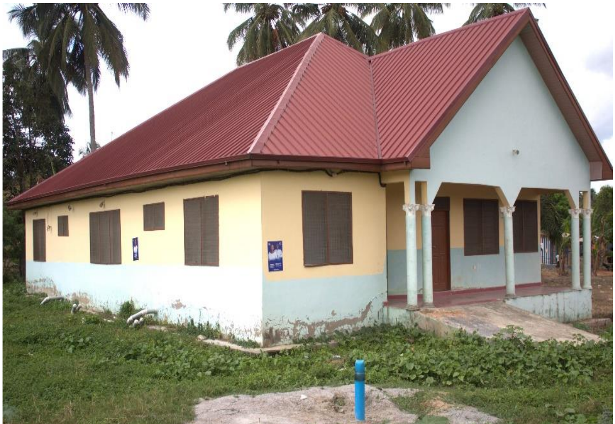
CONSTRUCTION OF CHPS COMPOUND AT DUOTO
