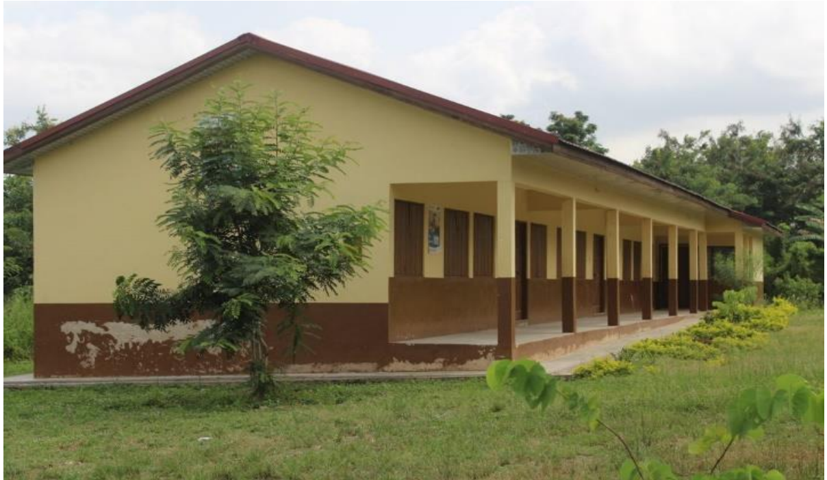
CONSTRUCTED 1 NO. 3 UNIT CLASSROOM BLOCK AT AG. TAWORA
