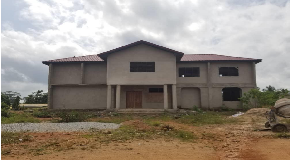
POLICE STATION AT AGONA NSABA
