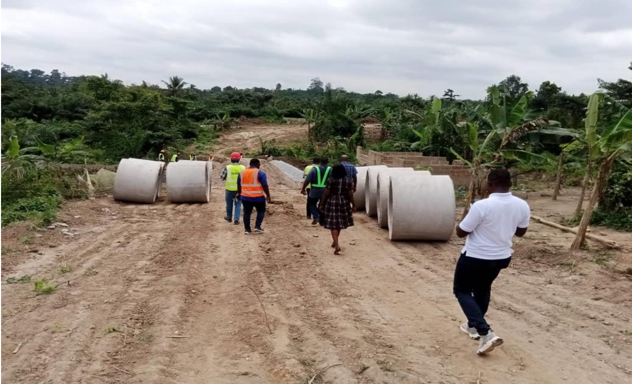
At Moree And 2no. 1200mm Diaiameter Pipe Culvert At Abura Dunkwa.
