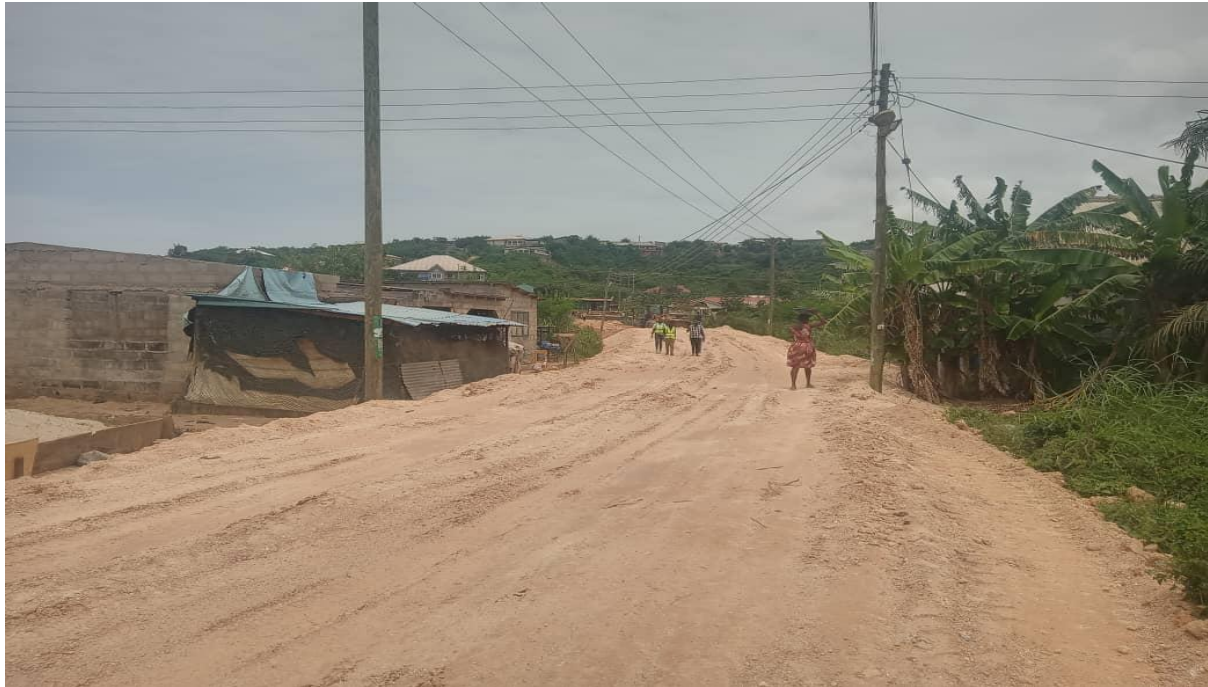
Reshaping of 130m Road At Tetsi, and 280m Road At Moree
