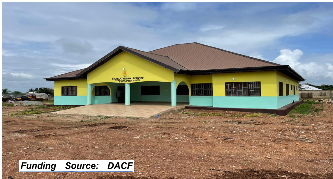
Key Achievement 1: Completed of a Health Center at Asuotiano
