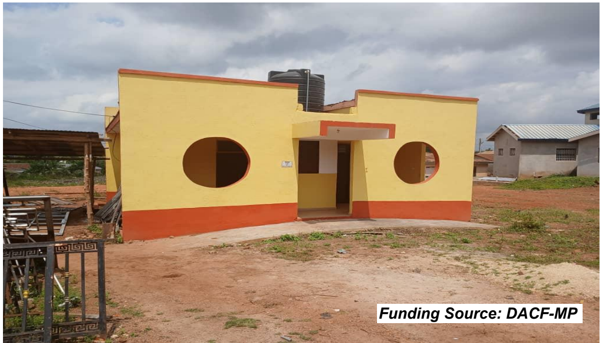
Key Achievement 3: Rehabilitated Toilet Facility at Asuotiano
