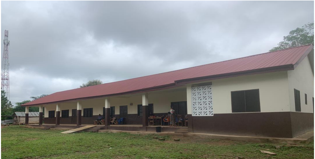
PICTURE 3: 1NO. 3 UNIT CLASSROOM BLOCK WITH AUXILIARY FACILITIES, STAFF COMMON ROOM AND STORES AT DOMFETE
