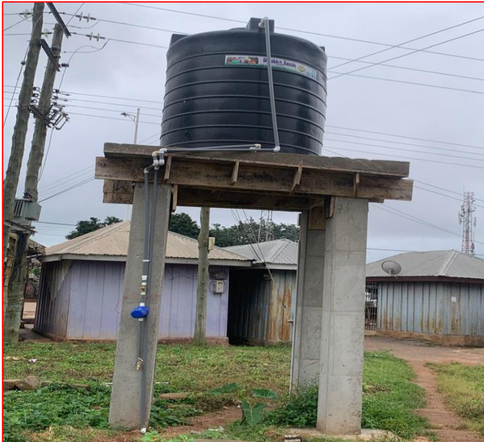
Drilled and mechanized of 1no. Borehole at Senase
