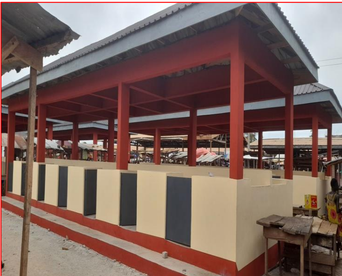
Completed 4no. 14-unit open market stalls at Thursday market
