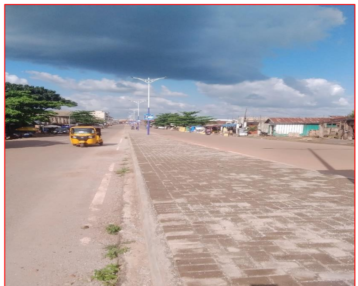
Street Lights and Pavements Constructed at Various Locations
