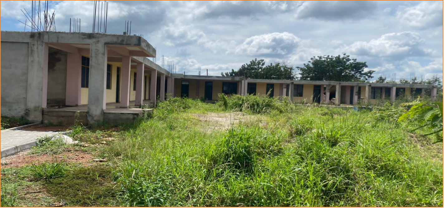
Constructed of 1no. Storey, 10units office complex block and external works at Berekum
