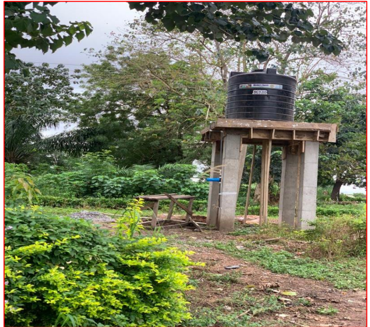
Drilled and mechanized of 1no. Borehole Continental
