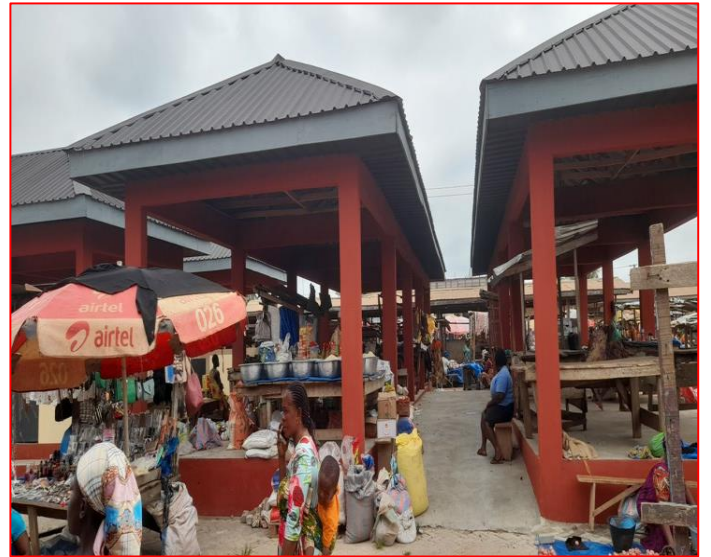
Completed 2no. Pavilion and paving of market access and market spaces at Berekum
