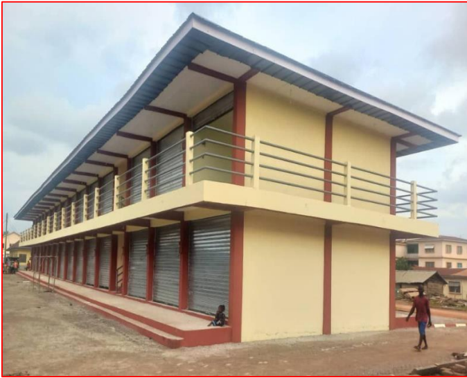
Completed 1no. 56unit lockable stores at Berekum Thursday Market Completed.
