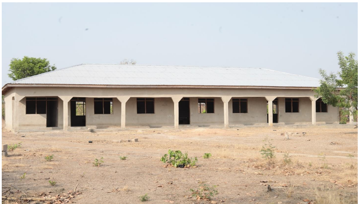
CONSTRUCTED CLASSROOM BLOCK OFFICE & STORE AT FAWOMAN ( DACF)
