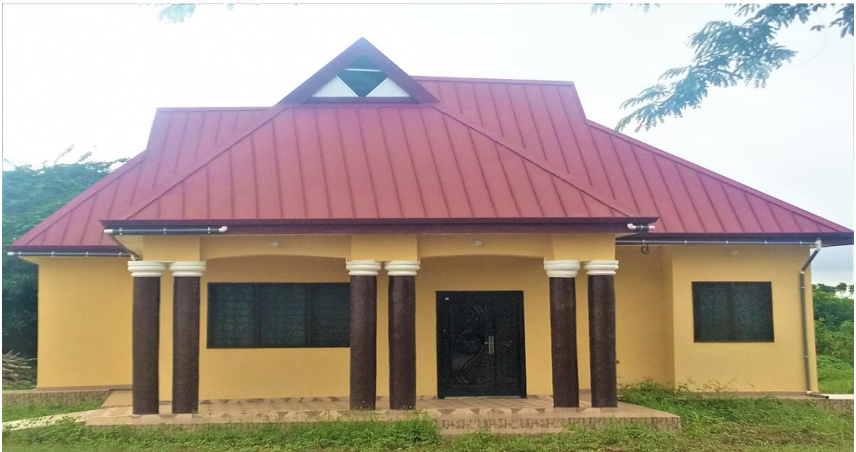
GES DIRECTORS BUNGALOW CONSTRUCTED
