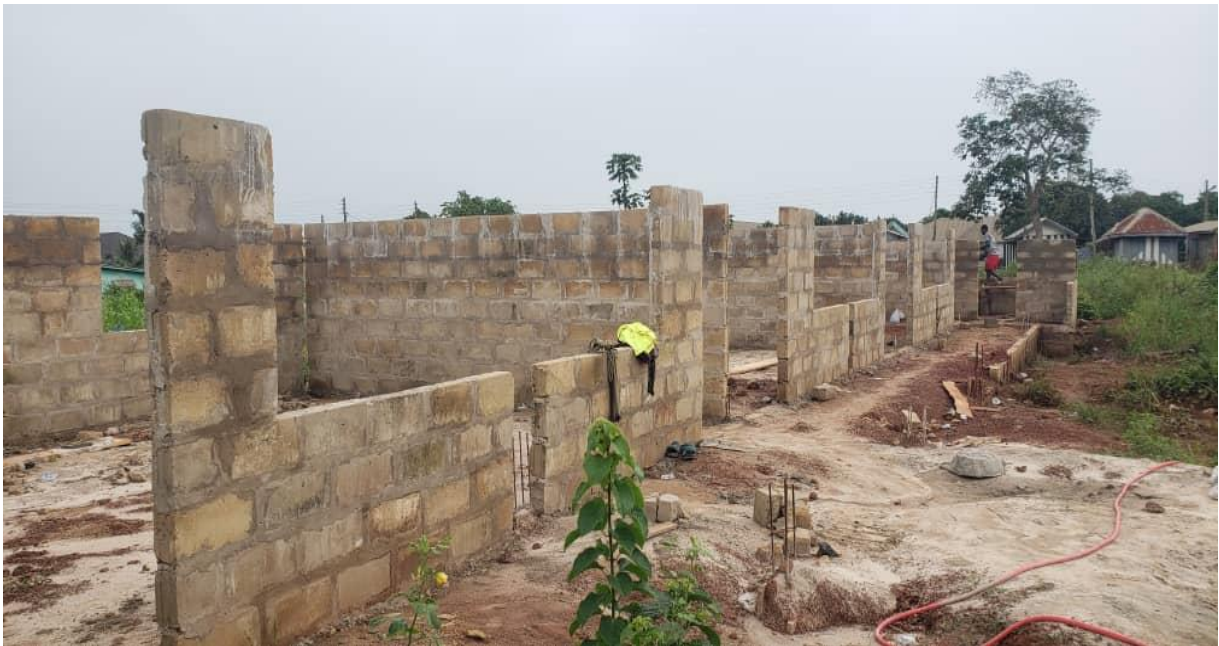
CONSTRUCTION OF 3 UNIT CLASSROOM BLOCK AT TUOBODOM MAGAZINE.
