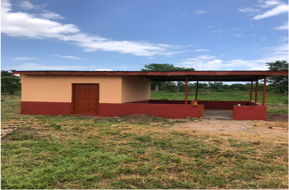
Completed 2No. Site Creches at Atrapa and Kwame Duro
