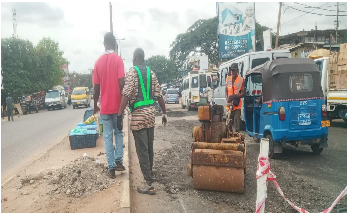
POTHOLE PATCHING ALONG SUAME-KRONUM HIGHWAY
