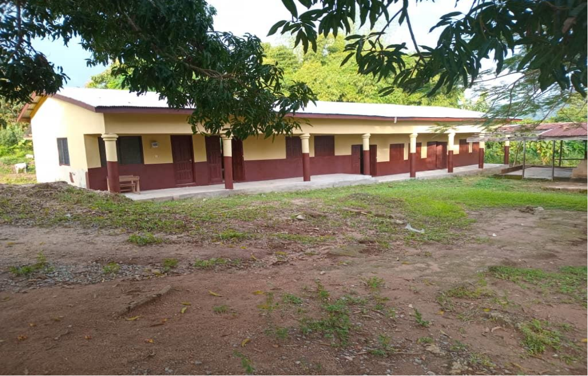
Figure 8: Construction of 1no. 3-unit classroom block at Adutwam – DDF
