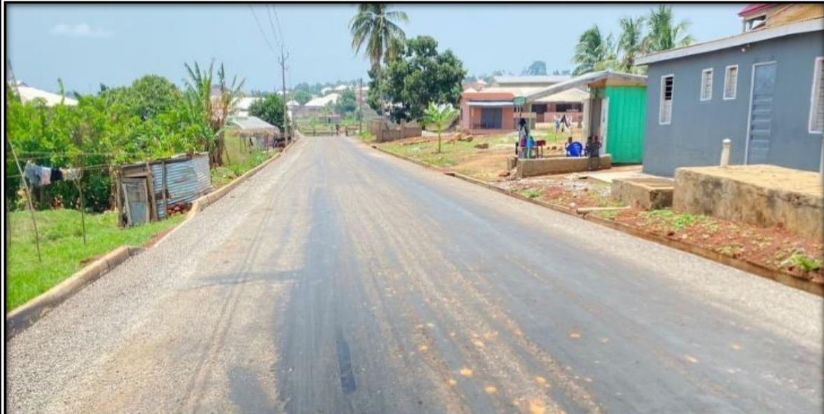
PROJECT DESCRIPTION: CONSTRUCTION OF ABRUKUTUASO 1.2KM (MR. ERNEST) ROAD LOCATION: MAMPONG
