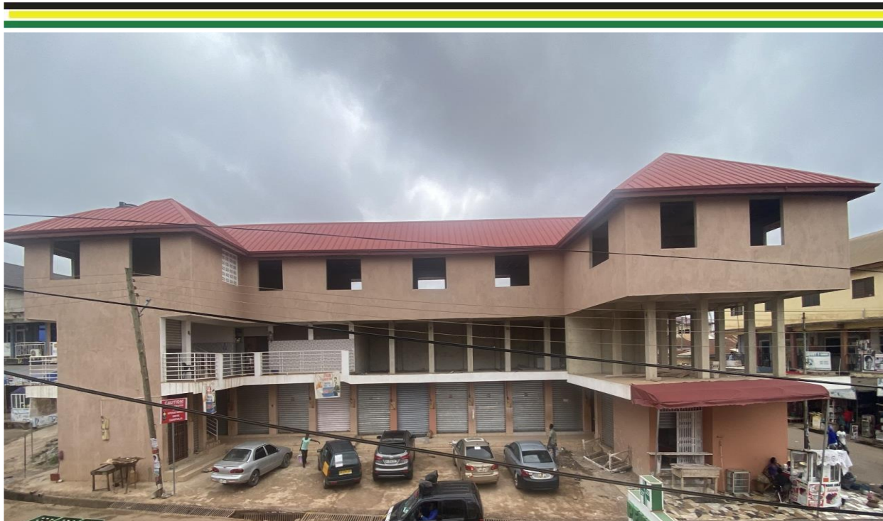
❑ ZONAL COUNCIL OFFICE CONSTRUCTED @ ATONSU (90%)
