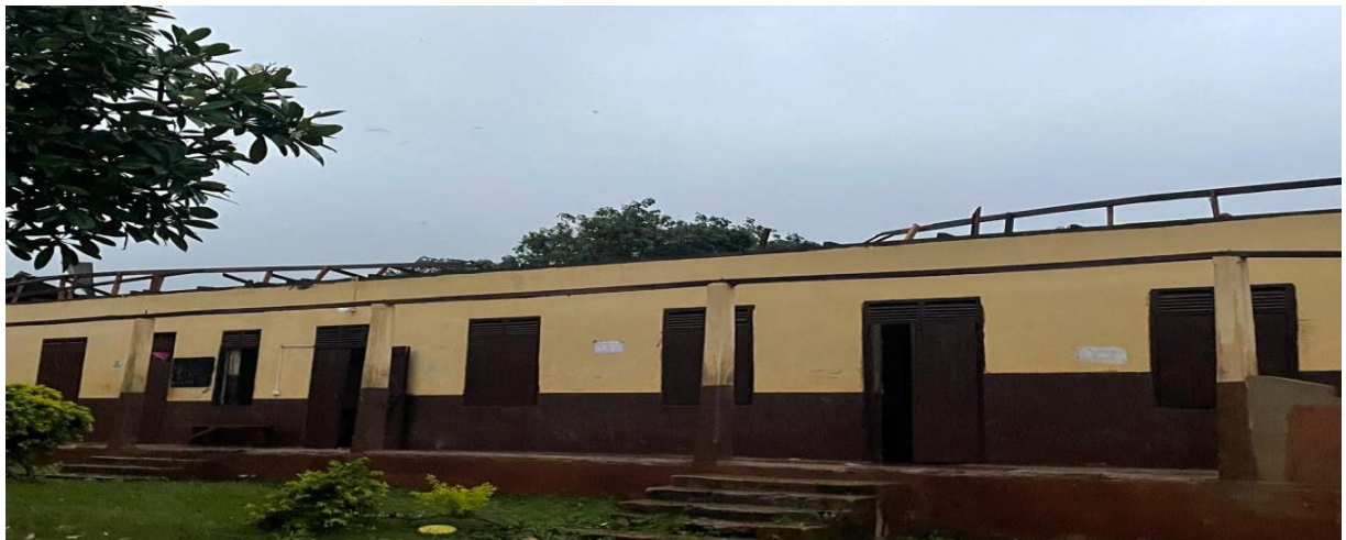
Rehabilitation of 1No. 3 -Unit Classroom block at Wioso)
