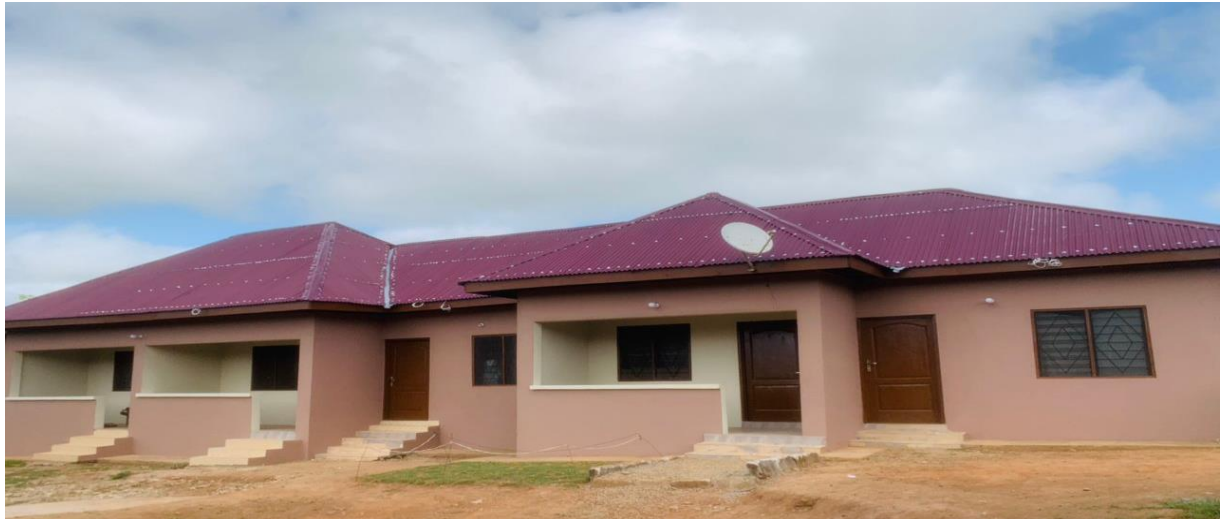
Completion of 1no 3-unit Chamber and Hall teacher's quarters at Adiembra
