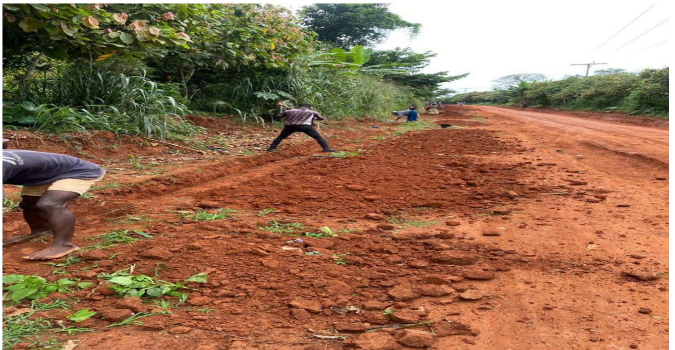
REHABILITATED 5KM ROADS AT SUNKWA, TENSO, ONWE AND DINKYIN
