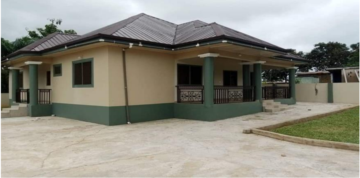
Completed 1No. 3bedroom Doctor's bungalow at Sankore FUNDING: Ghana Gas
