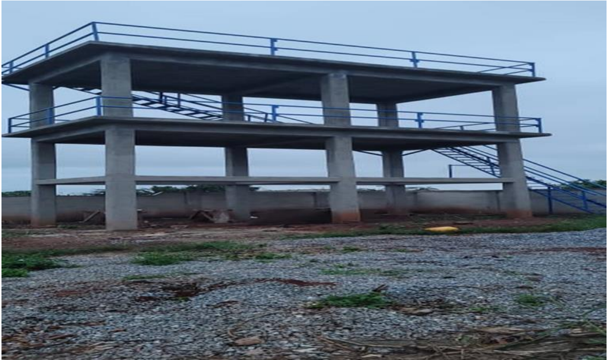
Completion of Small Town Water System- Noberkaw FUNDING -DACF/SWN
