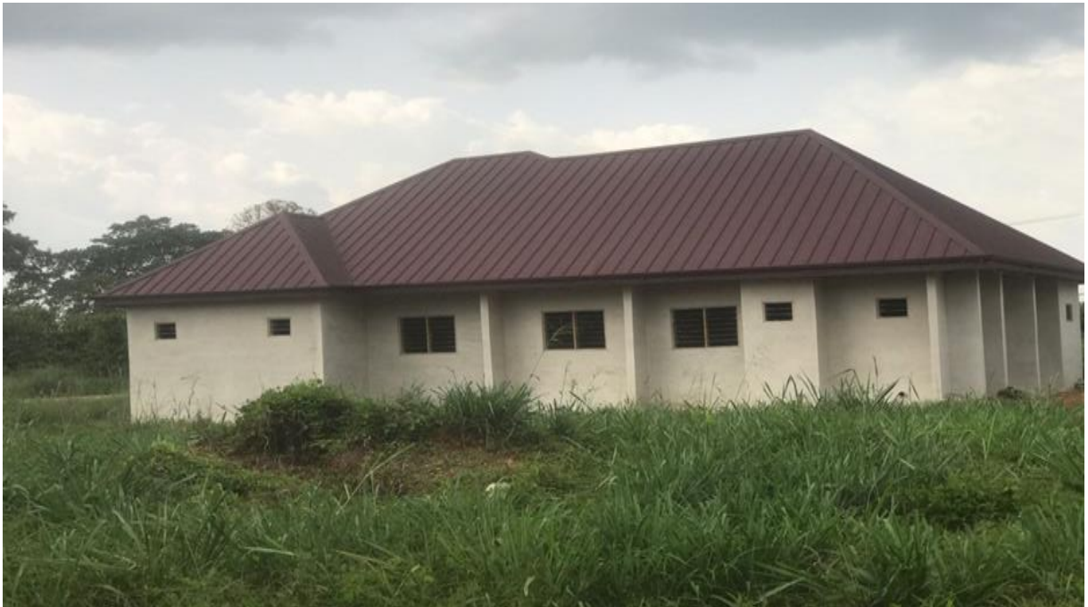
Completion of 1No. CHPS Compound at Amankwaakrom - On-Going FUNDING: JICA
