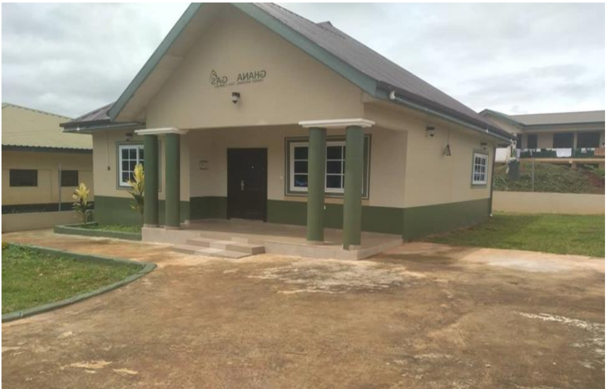
Completed 1No. 2-bedroom master's bungalow – Kukuom SHS FUNDING: Ghana Gas
