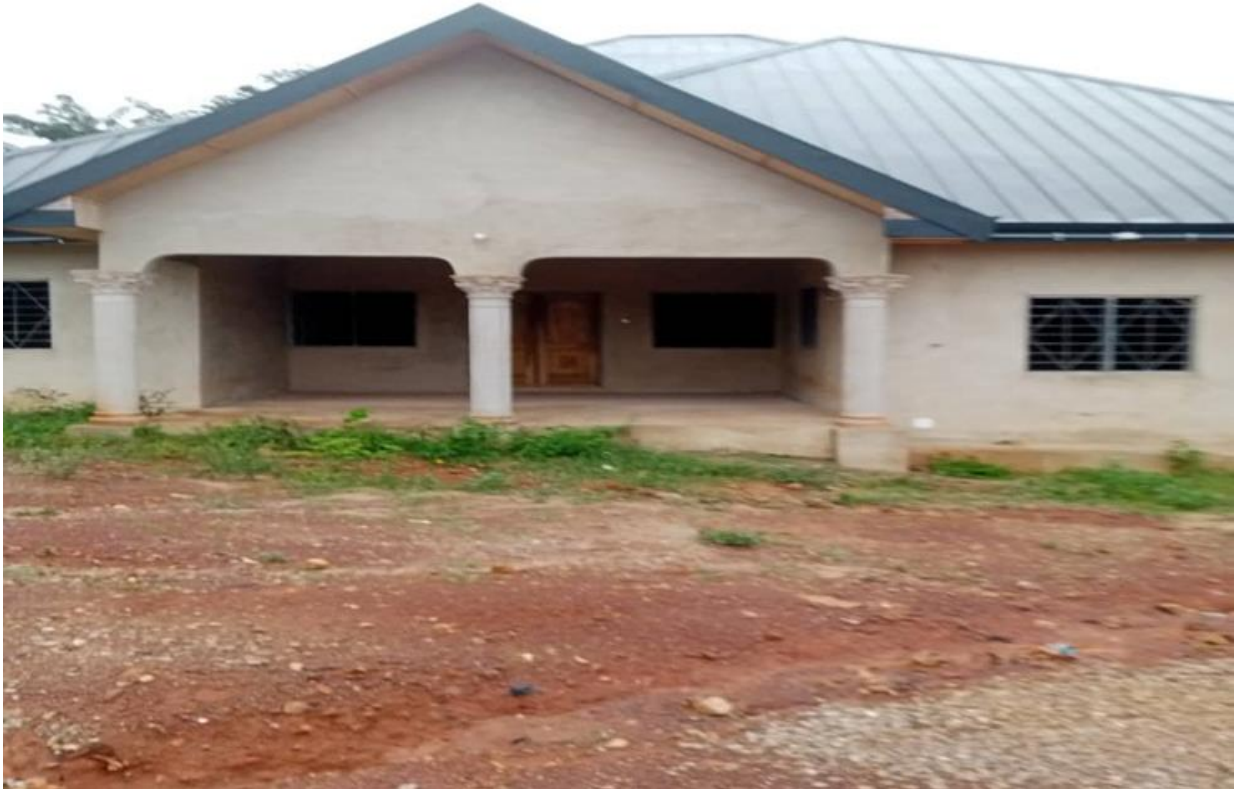
Completion of Police headquarters – Sankore FUNDING DACF Reserve Fund
