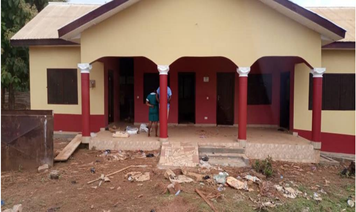
Completion of 1 No CHPS Compound – Asarekrom FUNDING: MPHf
