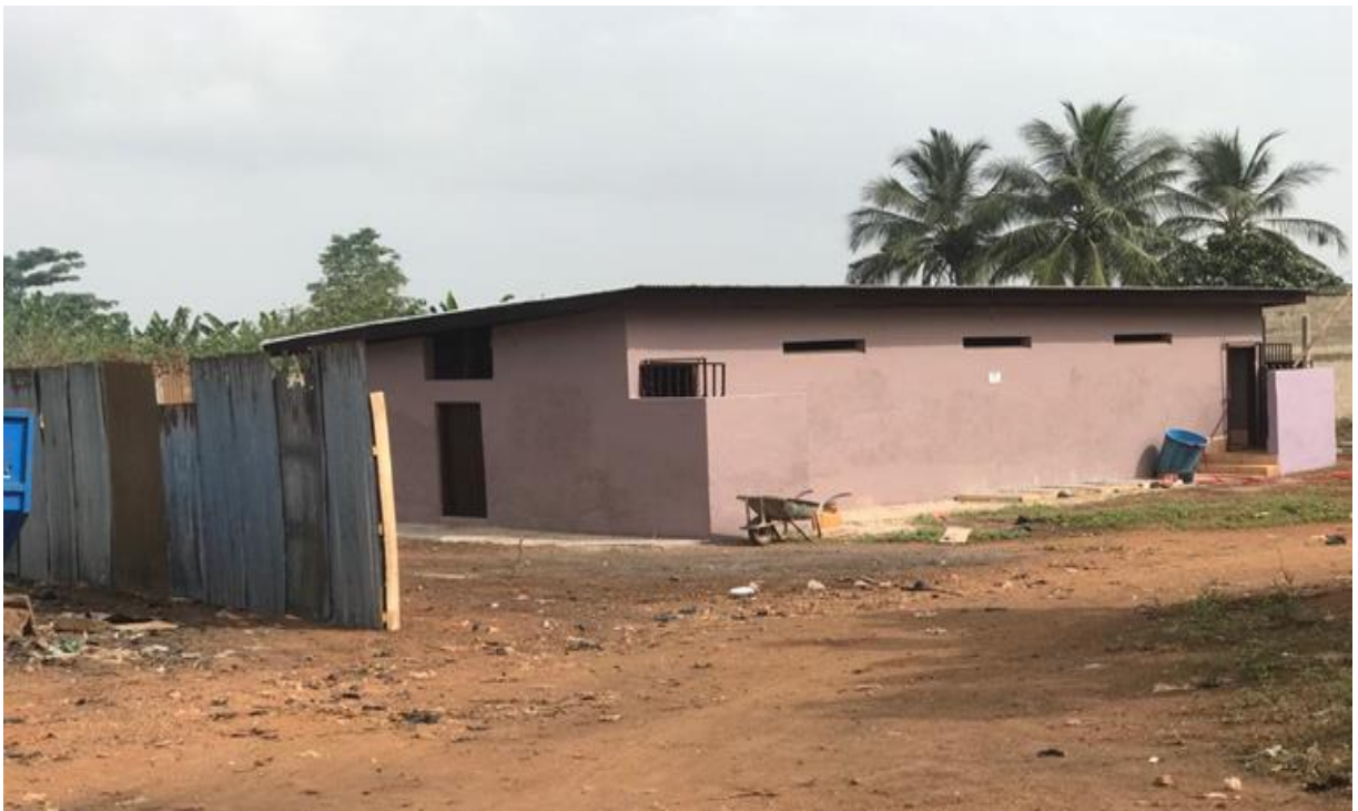
Renovated 1No. 12-Seater Aqua Privy Toilet at Kukuom FUNDING IGF
