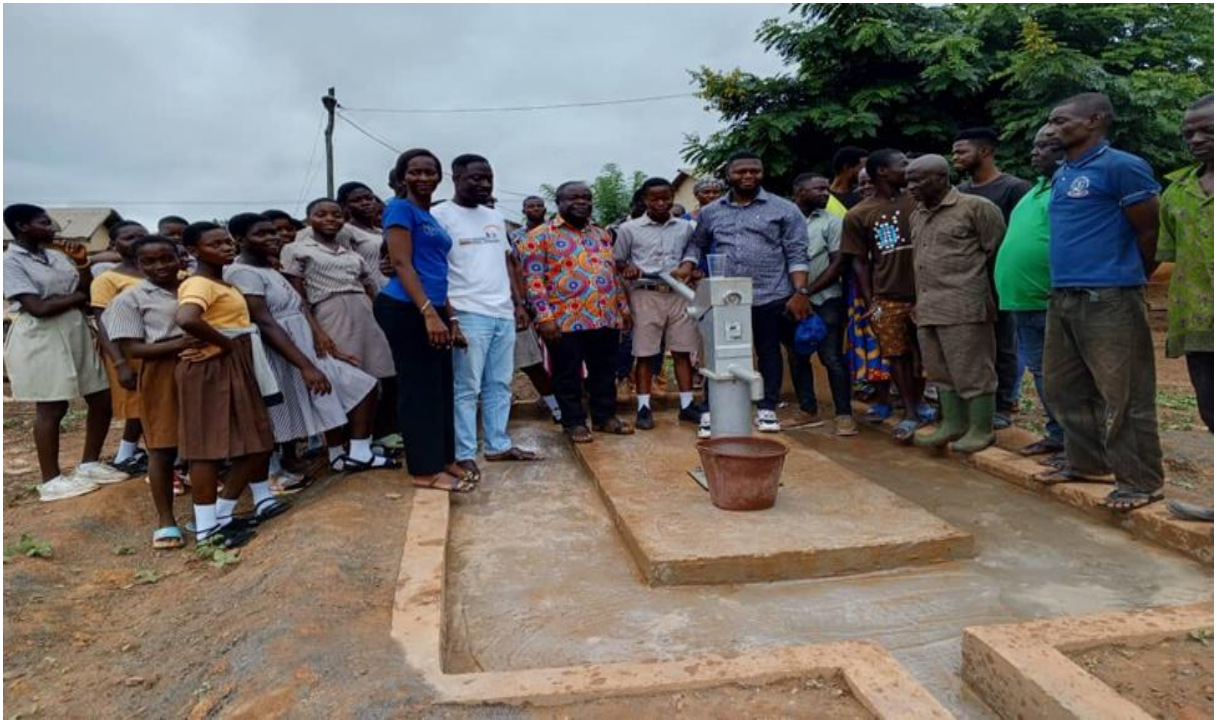
Mechanized 1No.2 Boreholes with Hand pump at Kwadoma and Pafu FUNDING: DACF
