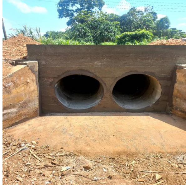
Construction of 1No. 1200mm \Theta concrete pipe Culvert on Bob Marley Road at Peki-Avetile (DACF-RFG)
