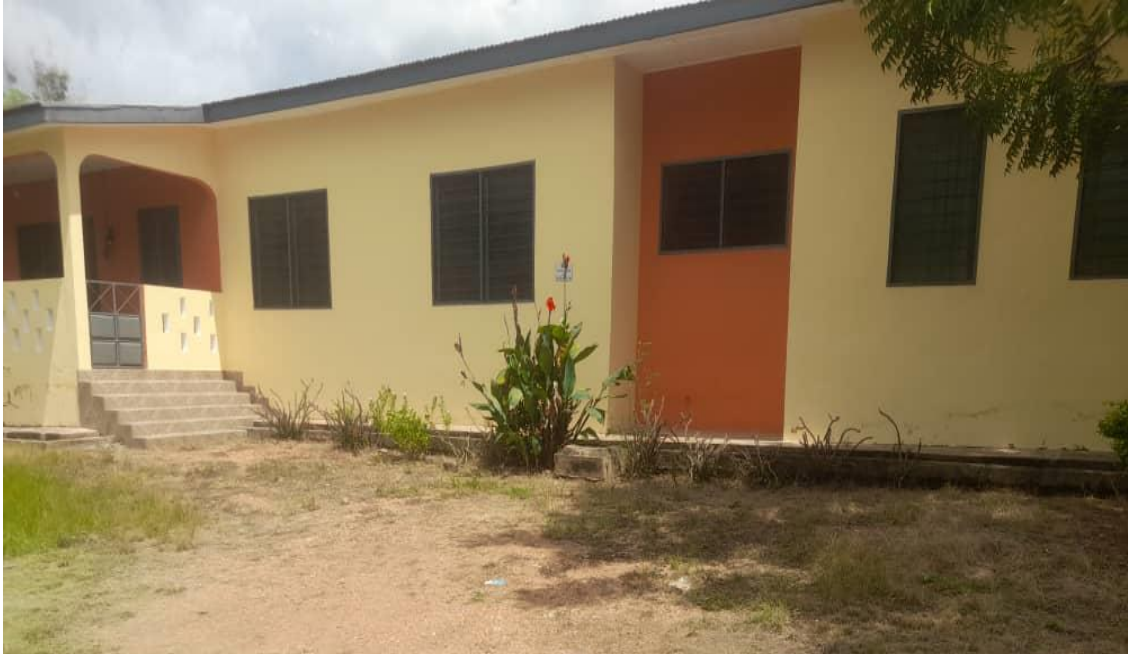
Renovation of DCD's Bungalow- (DACF)
