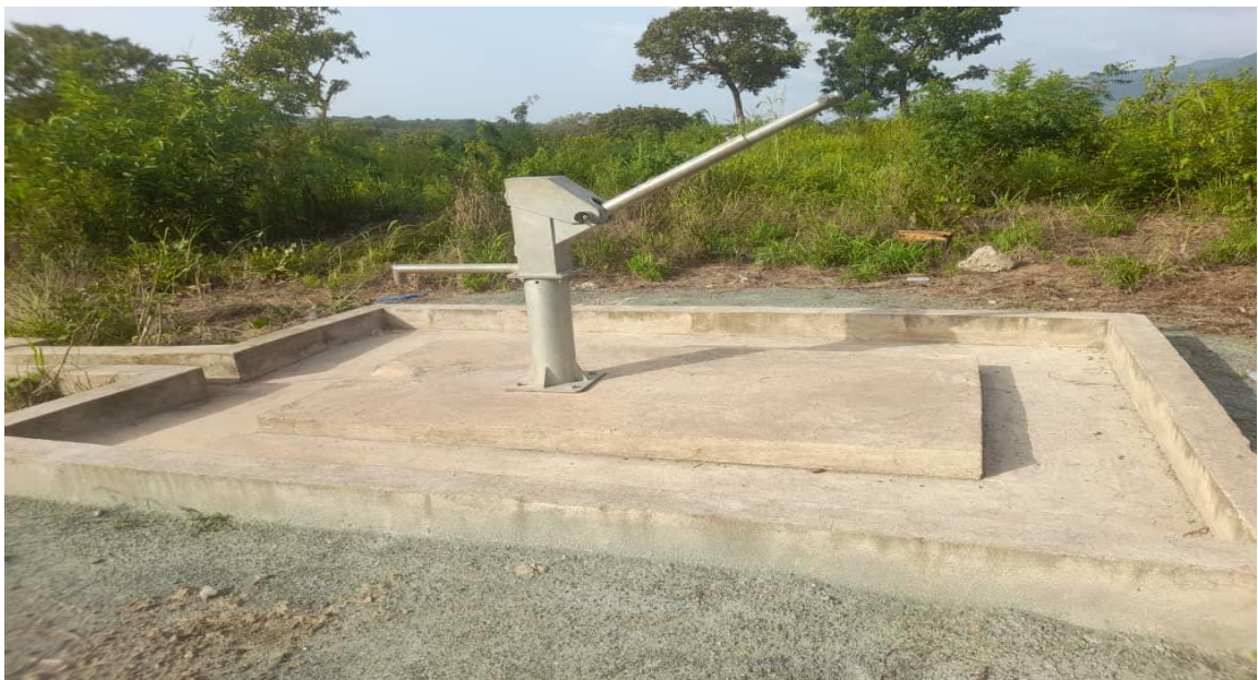
Completion of 5No. Boreholes- (DACF)
