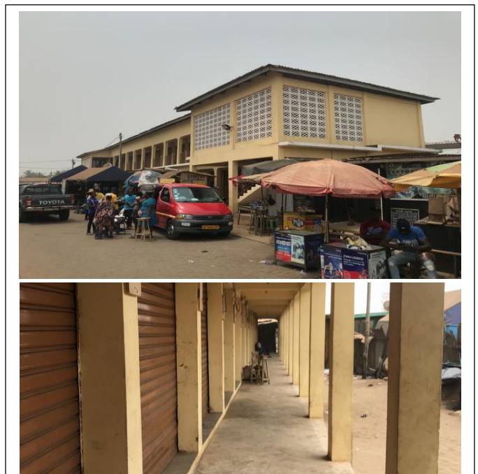
Completion of 28-unit lockable market stores at Aflao Lorry Park
