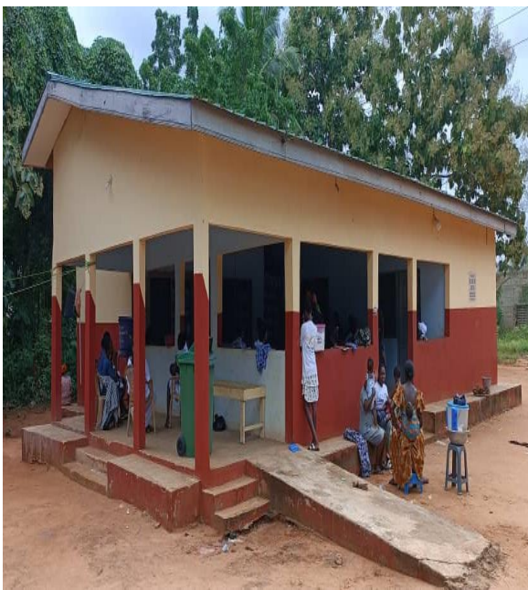
Completion of CHPS compound at Wudoaba
