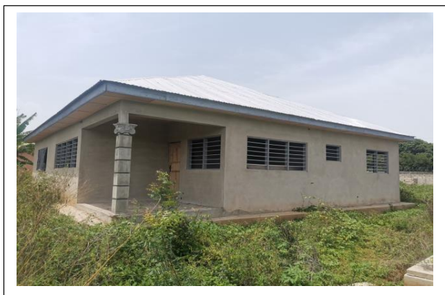
Construction of shelter home at Tokor
