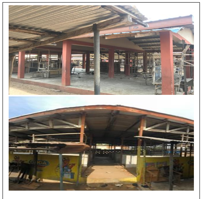
Denu market sheds renovated
