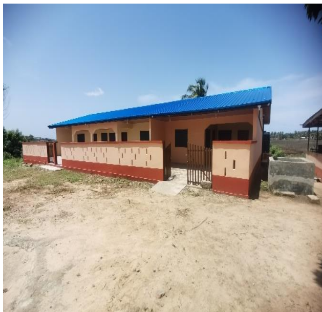
Completion of CHPS Compound at Wudoaba
