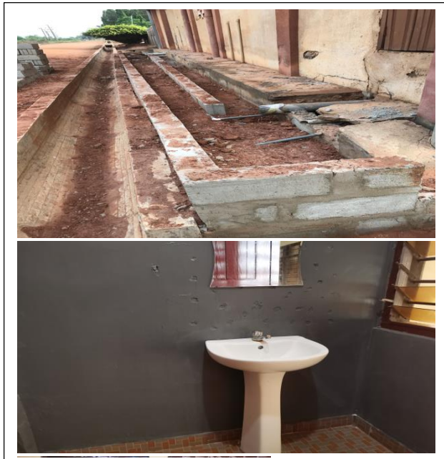
Office washrooms and drainage system were renovated
