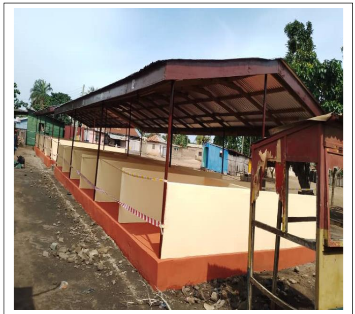
Aflao- Avoeme Market Shed renovated
