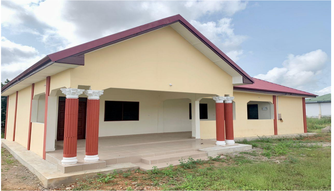
Canteen facility around Ho Municipal Hospital (DACF-RFG)
