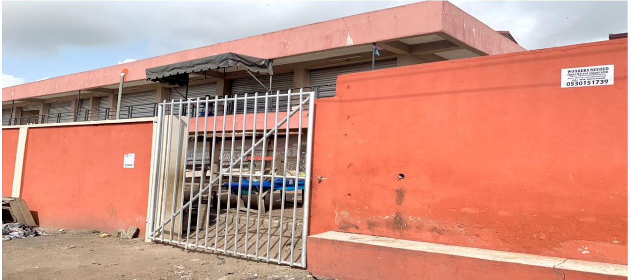
Fence wall around Ho Central Market (IGF)
