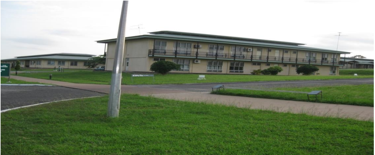
Figure 2: Regional Hospital - Ho
