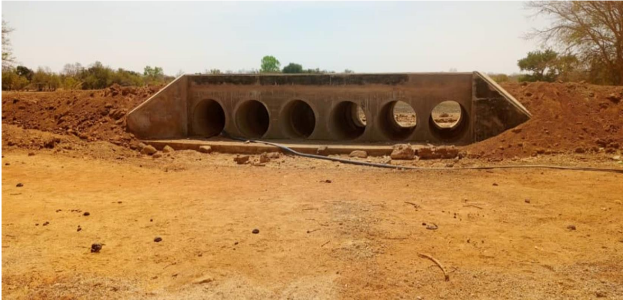
Constructed of 1 No. 6 No. Cell 1.2m pipes culvert at Kajelo
