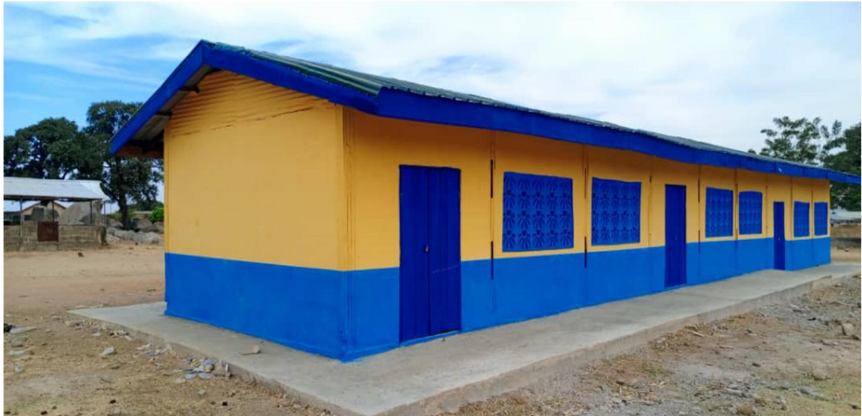
Constructed 1 No. 10 Seater Water Closet Toilet Facility at Paga Market
