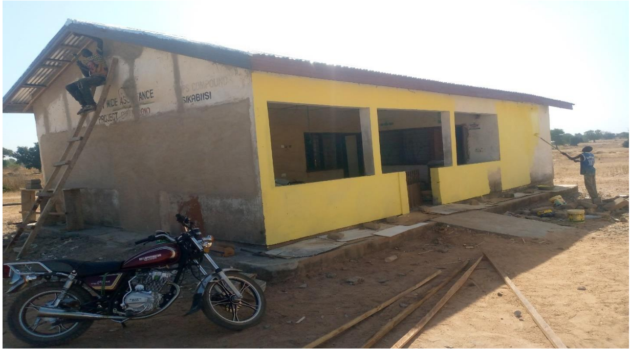
Refurbishment of Sikabiisi CHPS Compound
