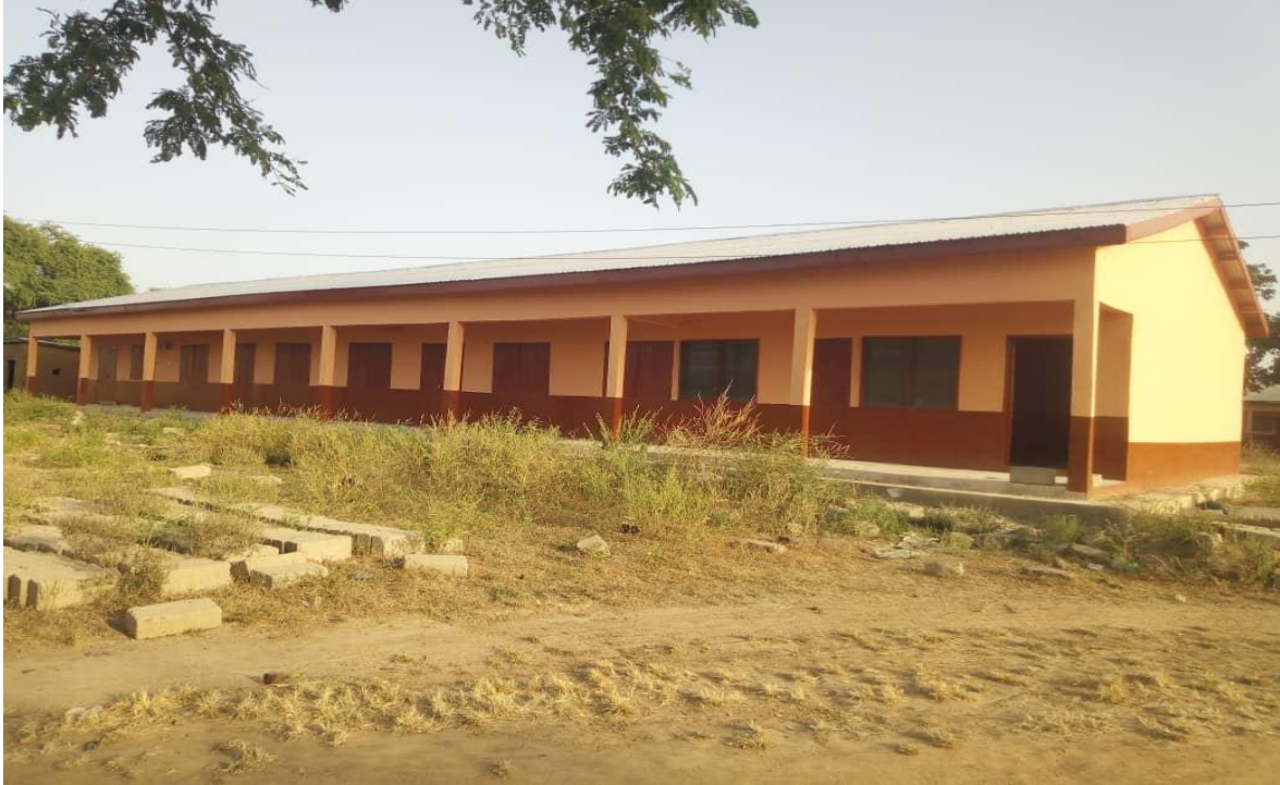
Construction of 3-Unit classroom Block with Ancillary Facilities at Kansoe
