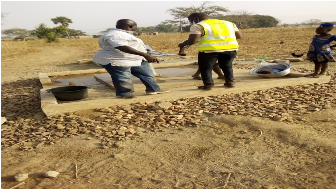
Drilling and construction of 20 No. boreholes (DACF-RFG)
