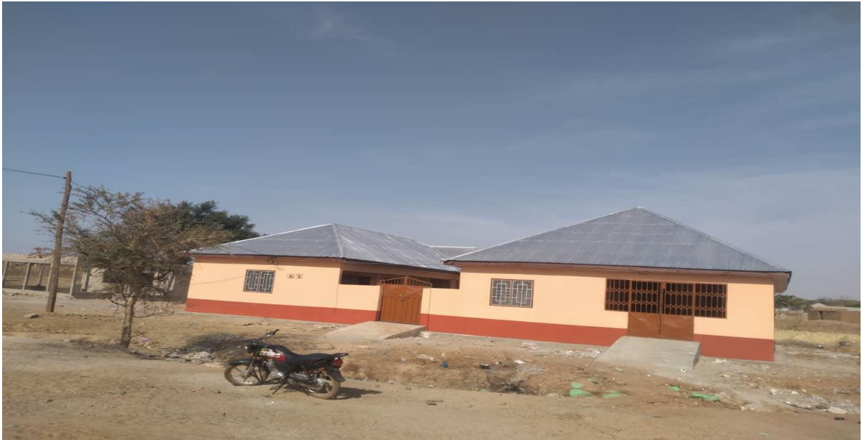
Construction of 1No.CHPS Compound at Kpalugu with furniture
