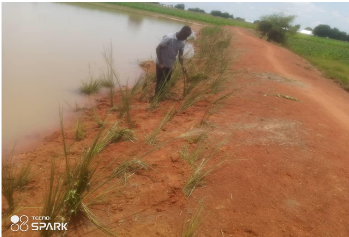
Planting of vetiver grasses to protect dam wall at Tempelim
