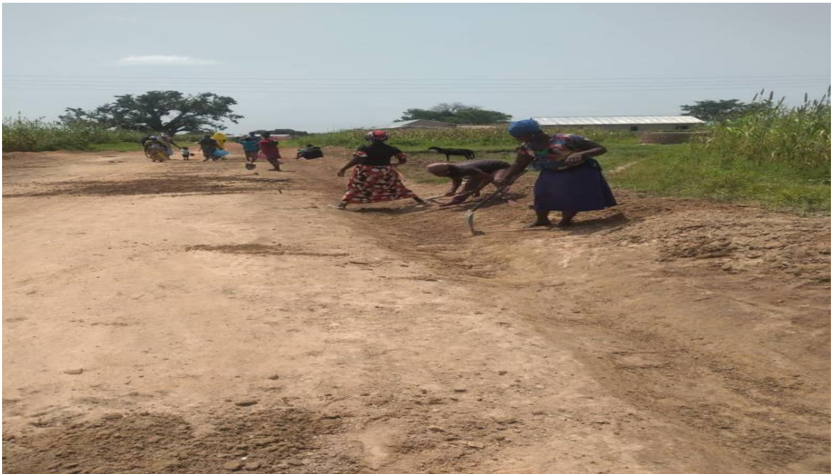
Rehabilitation of Nayoko No.2 - Goore Clinic Feeder Road (5.5Km)
