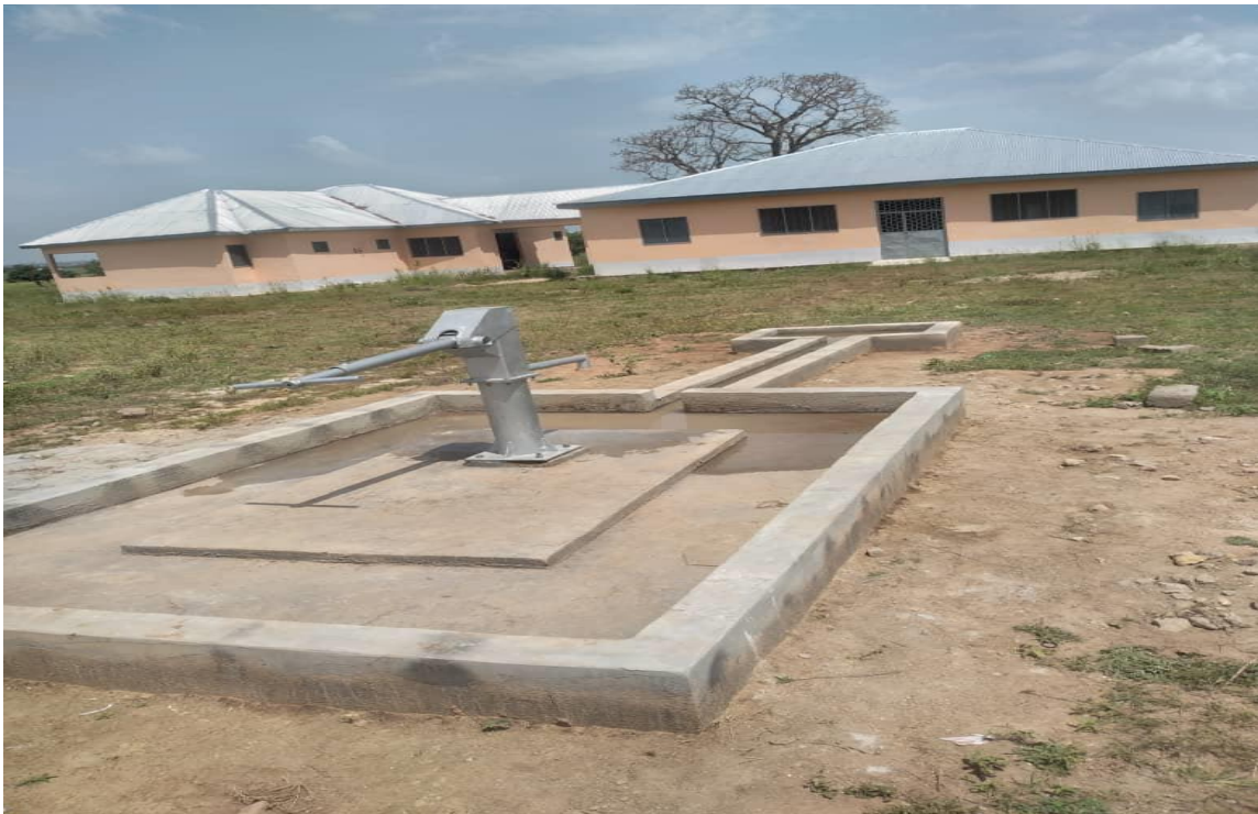
Drilling & Construction of 4No. Boreholes fitted with Hand Pumps at Bakanga, Barabogo, Manga, and Sakpari
