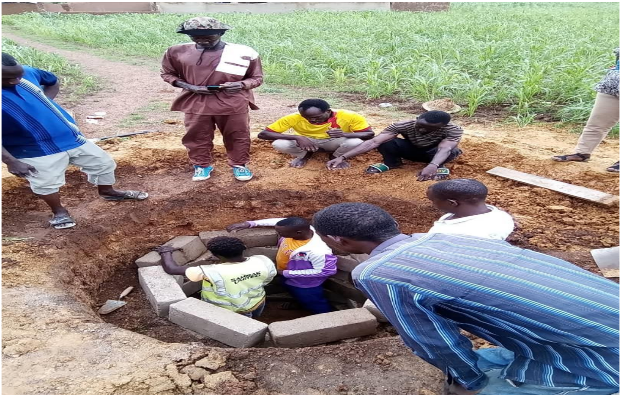
CLTS - Training of Artisans on Latrine Construction at Tegbilla
