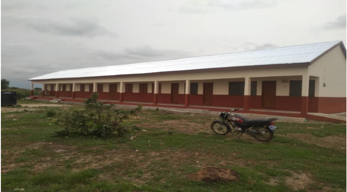
Construction of 1No. 3-unit classroom block at Belimpiisi with furniture
