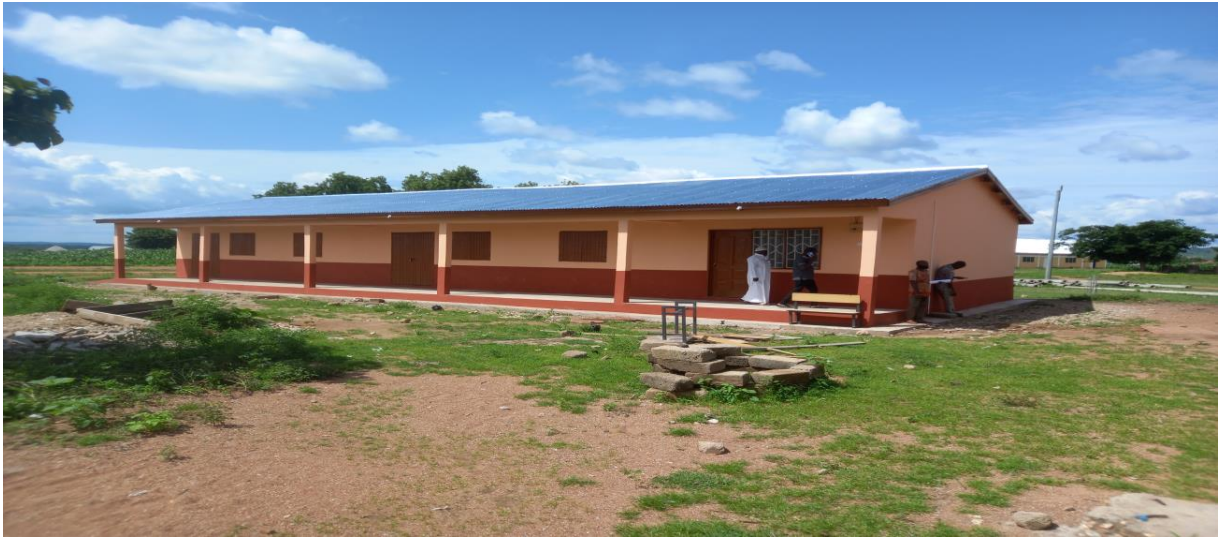
Construction of 1No. 2 Unit Classroom Block with office and store at Yalugu
