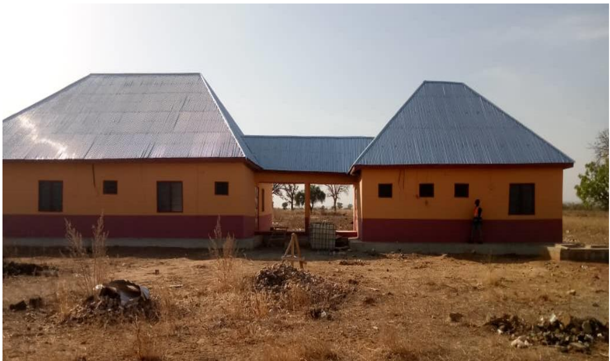
Picture 2: Constructed 1No.CHPS Facilities at KOBOUGU
