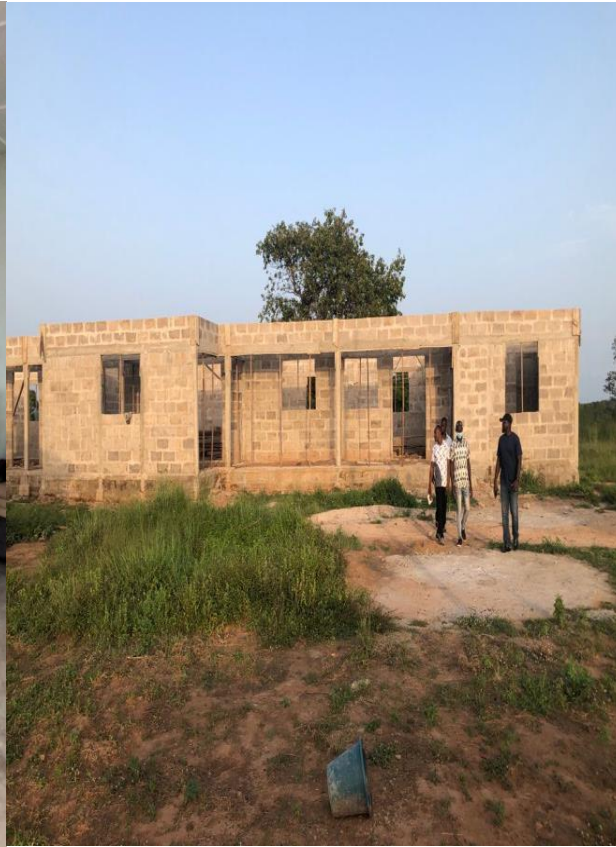
CONSTRUCTION OF 1 NO. 3 UNIT CLASSROOM AT SORI 2
