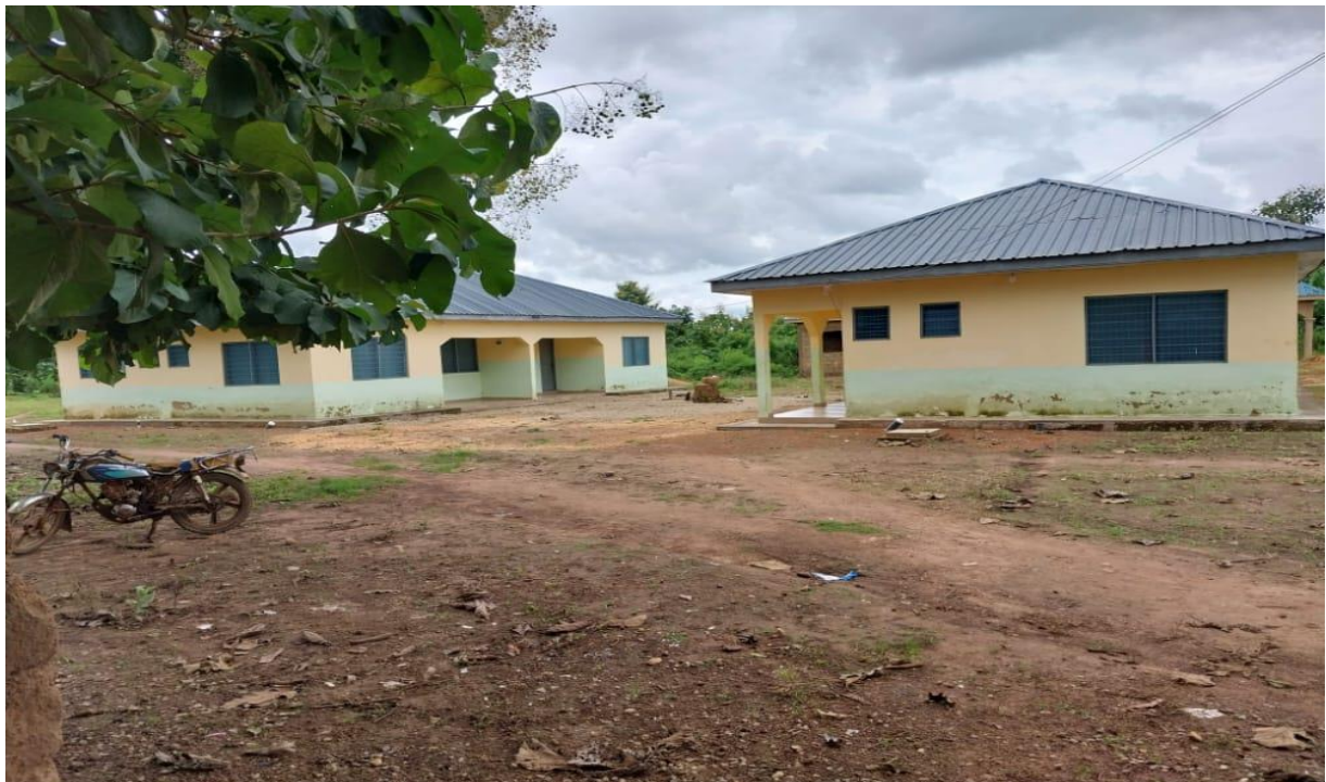
FINAL PAYMENT A CHPS COMPOUND COMPLETED AT ABUNYANYA
