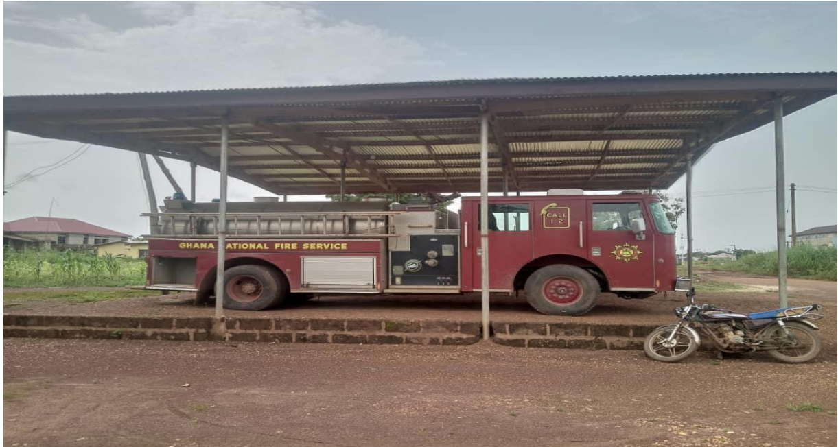
CONSTRUCTION OF FIRE SERVICE AND AMBULANCE BAY AT KPASSA
