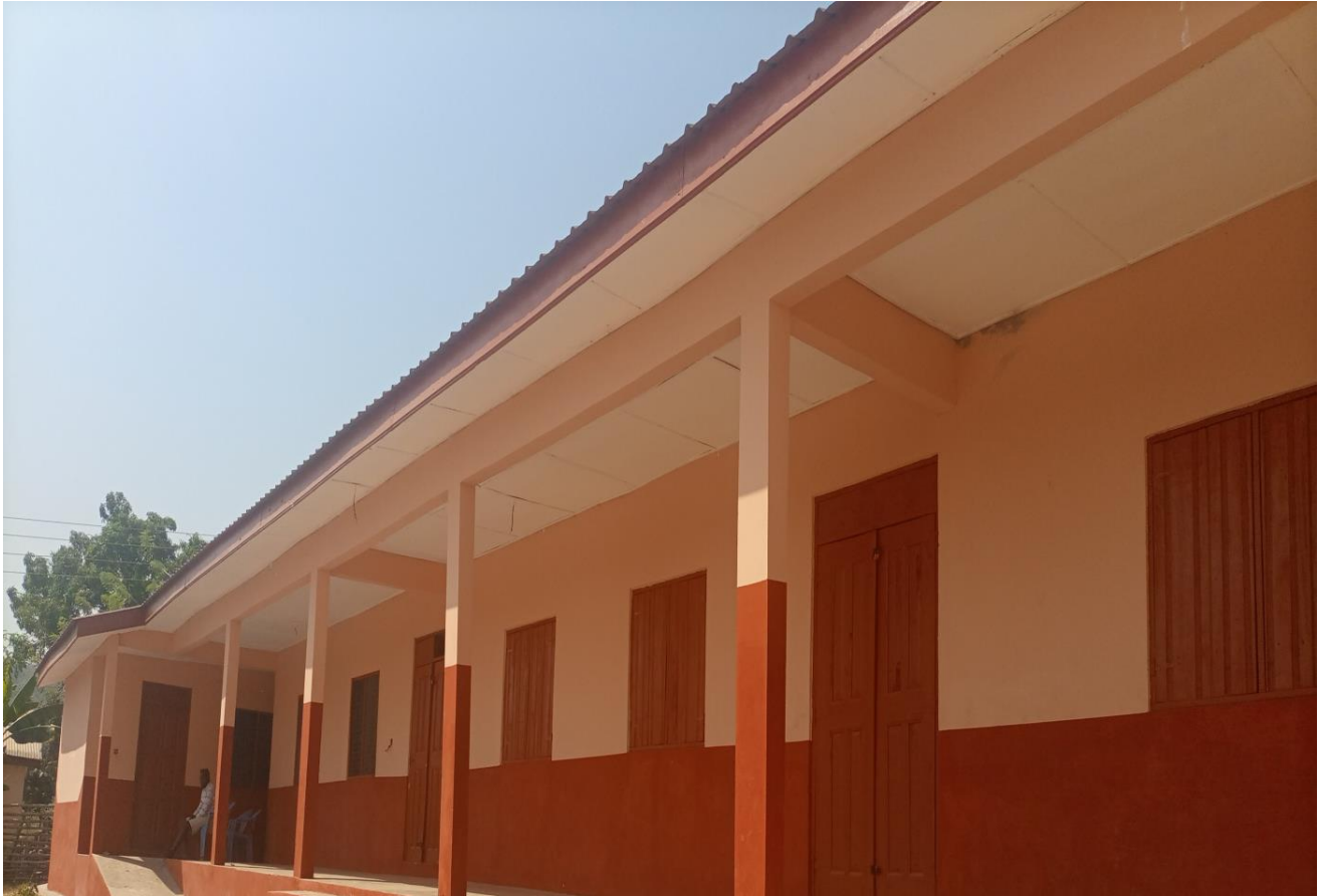
3-unit classroom block at Okanta
