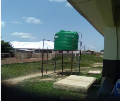
WATER STORAGE FACILITY AT DOHINI CLINIC
