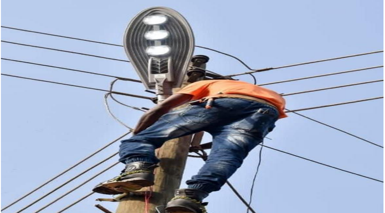
Fixing of streetlight
