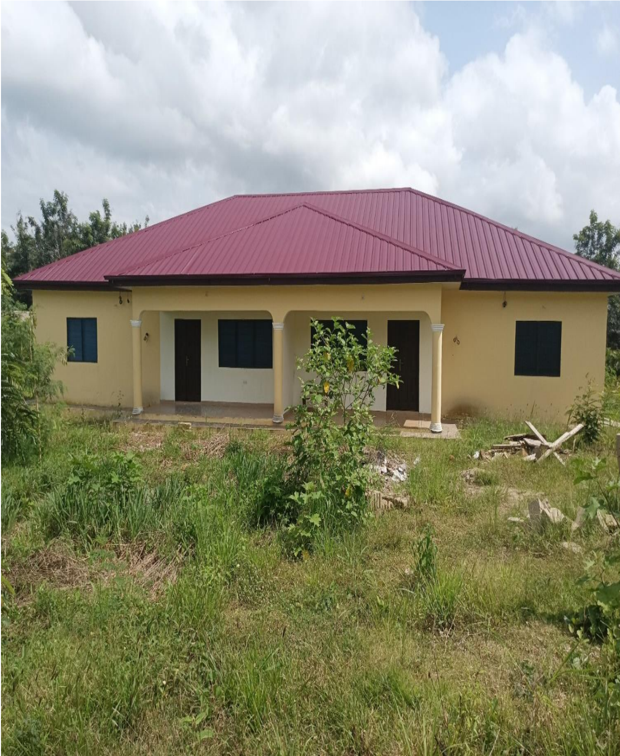
Picture 3: Construction of 1 No.2 Bedroom Teachers Bungalow at Potsin
