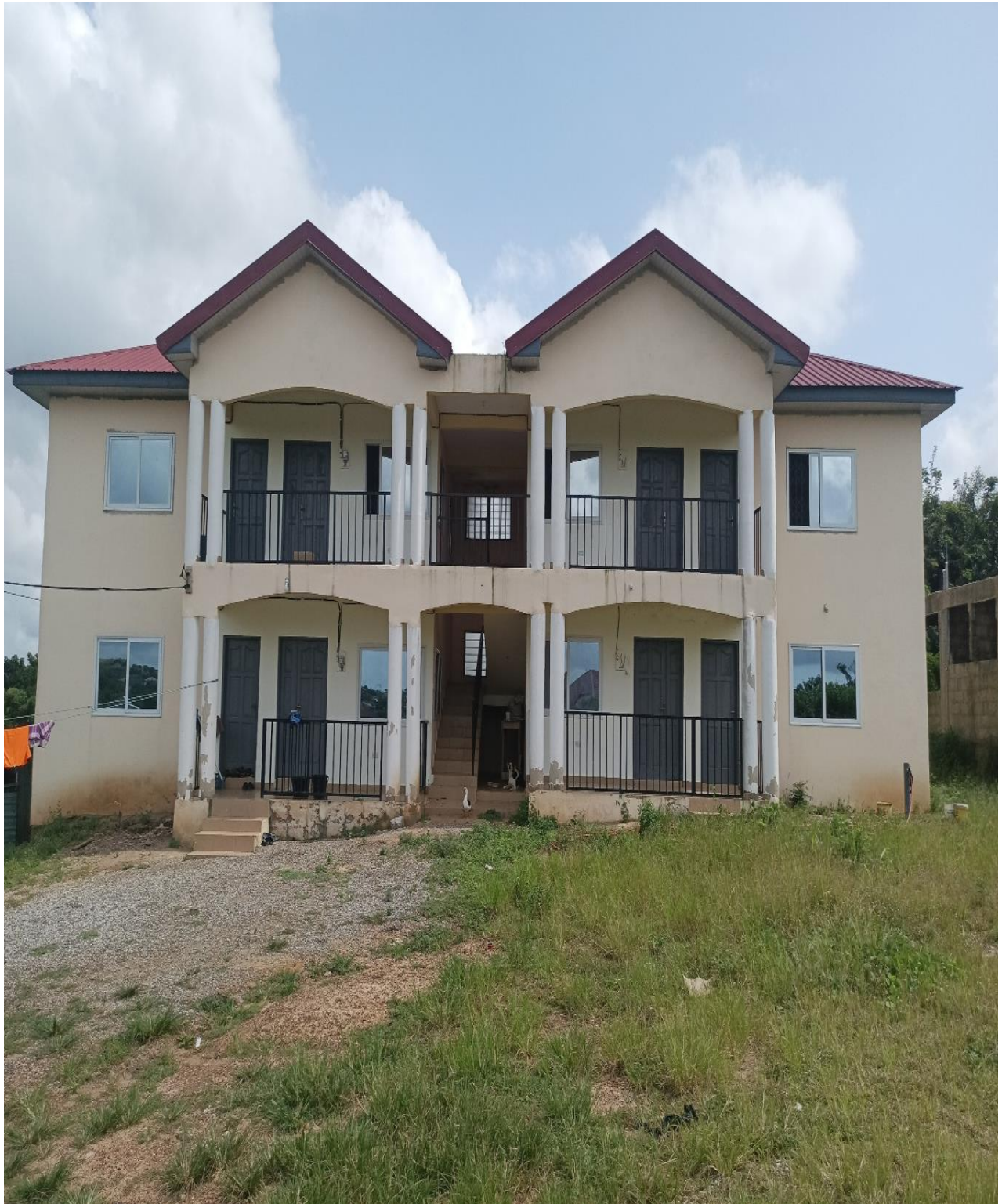
Figure 4: Construction of 1No 4. Semi-Detached bungalows for nurses in Gomoa
